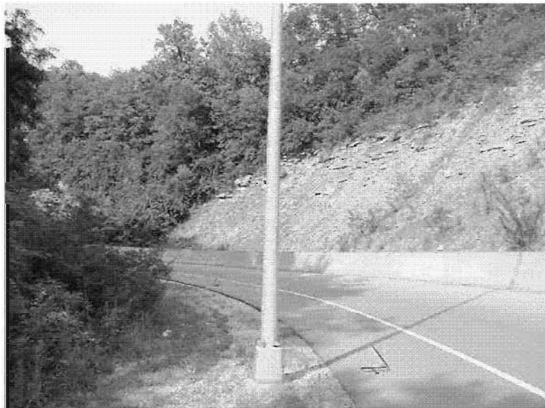
Figure F-32: HAM-71-10, moderate hazard potential (96)
