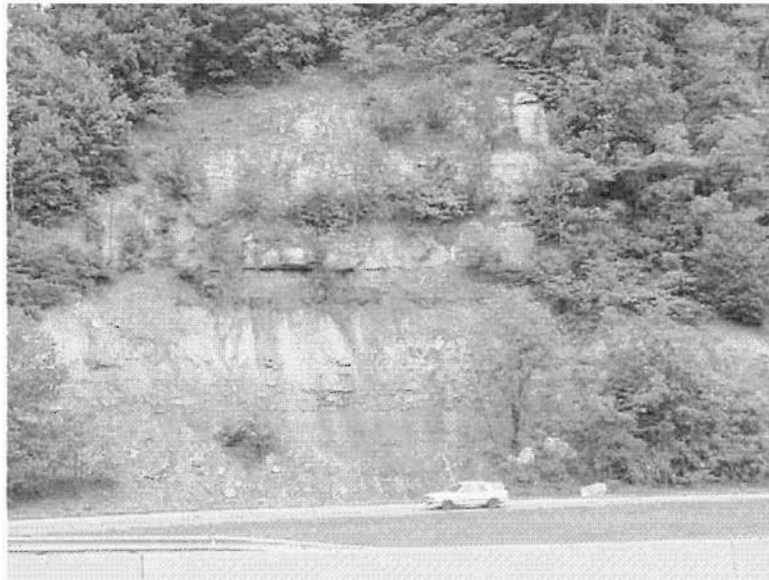
Figure F-24: COL-7-3.3, high hazard potential (103)
