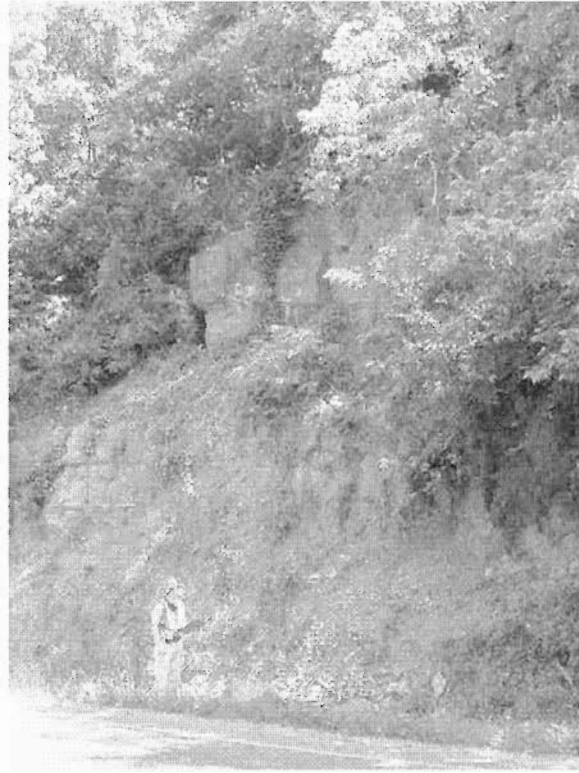
Figure F-21: GAL-160-0.55, high hazard potential (108)
