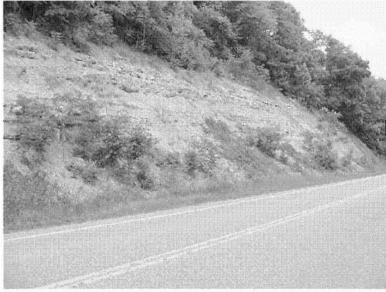
Figure F-81: ATH-78-2.25, moderate hazard potential (58)
