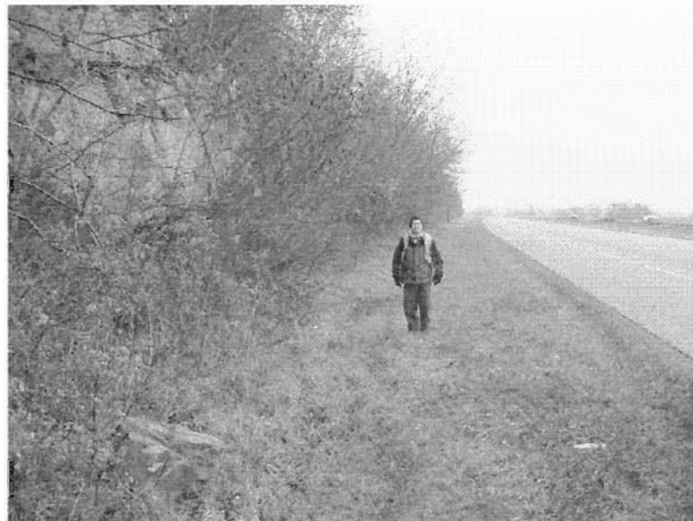
Figure F-108: COL-7-1.5, low hazard potential (23)
