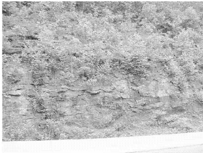
Figure F-18: JEF-7-33.3c, high hazard potential (111)
