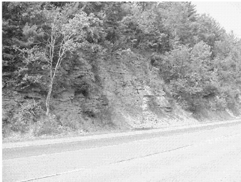
Figure F-67: LIC-70-135, moderate hazard potential (71)
