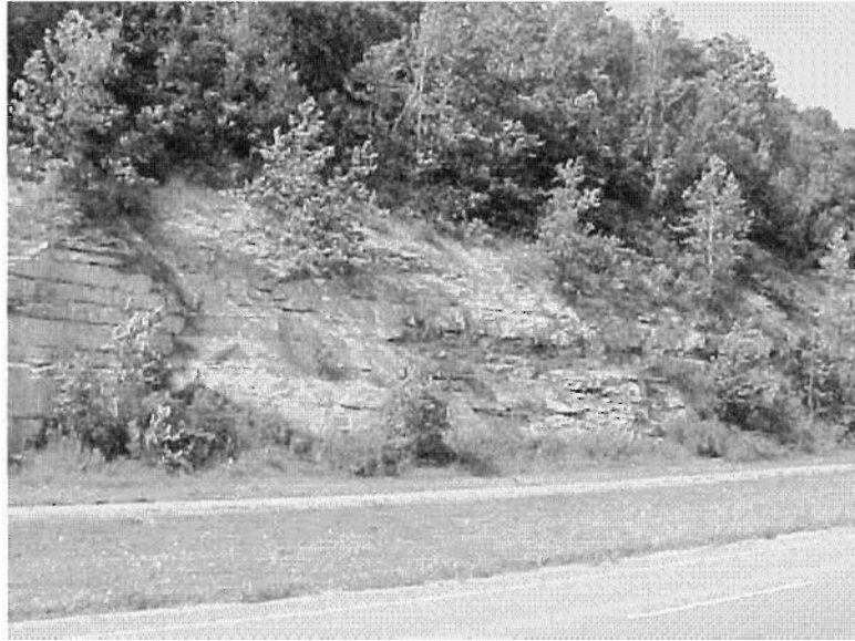
Figure F-79: COS-36-28, moderate hazard potential (60)
