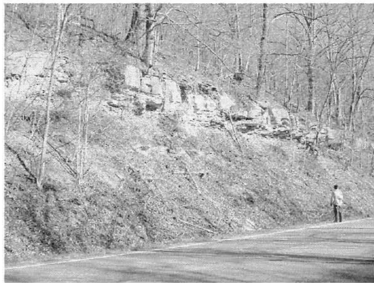
Figure F-2: COL-170-13.5, high hazard potential (146)
