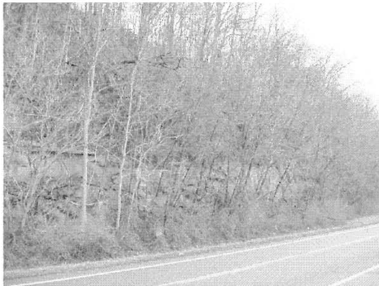
Figure F-103: WAS-7-36.5, low hazard potential (37)
