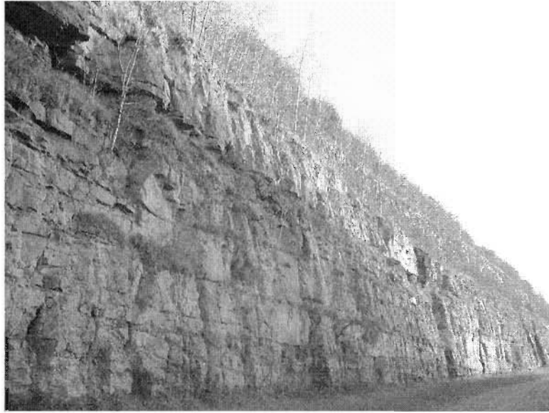
Figure F-51: TUS-77-63, moderate hazard potential (82)
