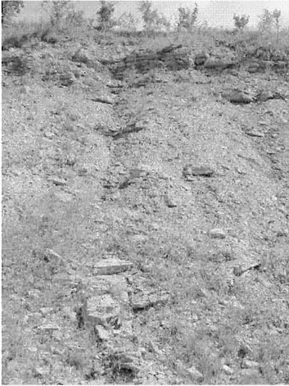
Figure F-29: HAM-74-17.6, moderate hazard potential (97)
