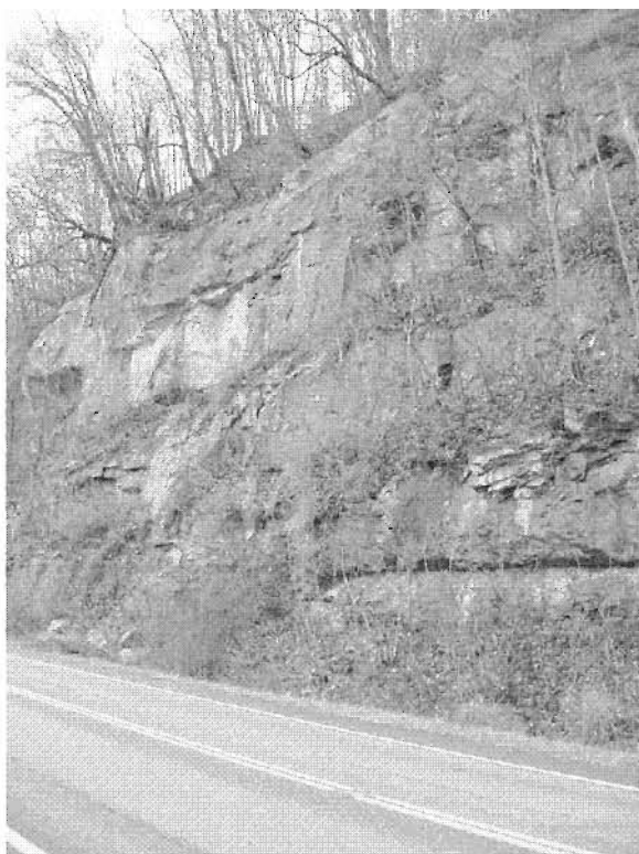
Figure F-12: WAS-7-39.5, high hazard potential (119)
