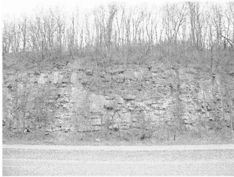
Figure F-31: TUS-250-23, moderate hazard potential (97)
