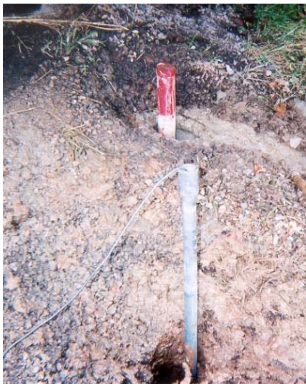
Figure 3.12 - Installation of TDR Cable Using 1.5 in (3.8 cm) Diameter PVC Pipe
