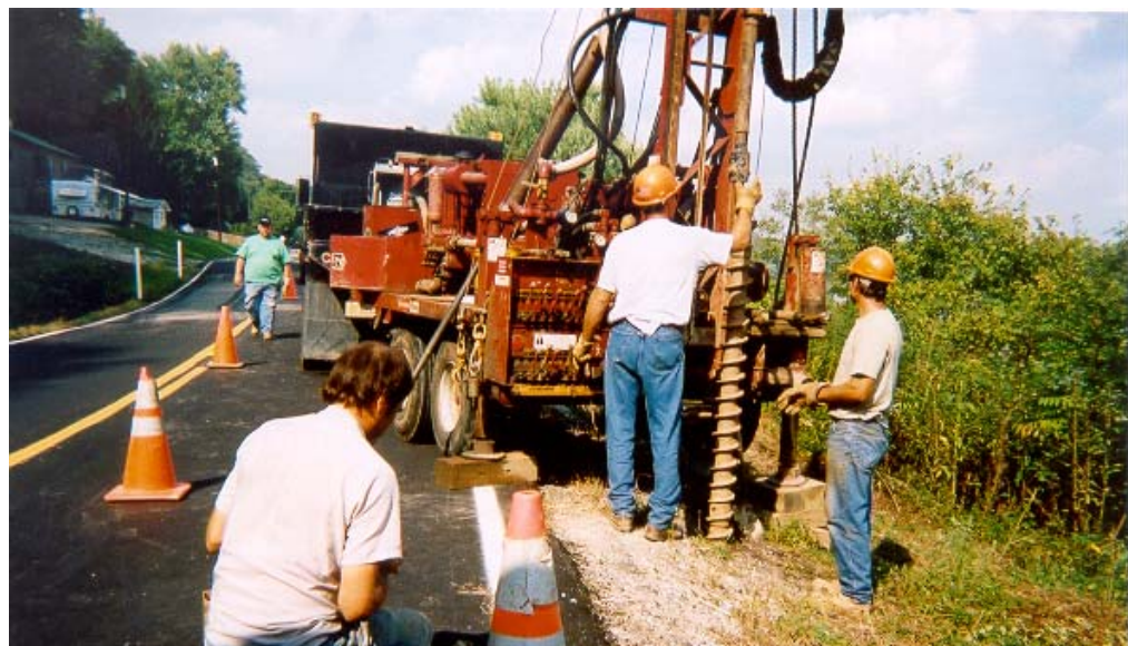
Figure 3.6 - Installation of Instrumentation at MEG-124 Site
