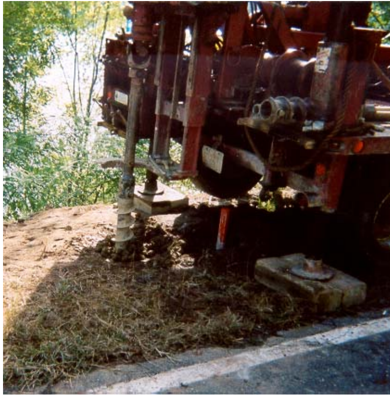
Figure 3.11 - Drilling TDR Boring Adjacent to Inclinometer Installation at MEG-338 Site
