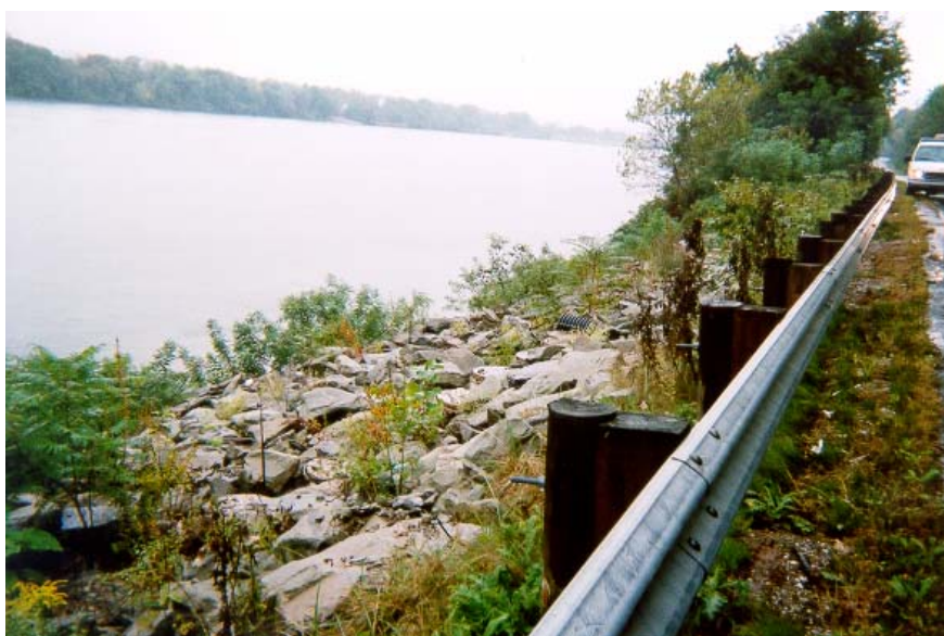
Figure 3.2 - Stabilized Rock Embankment along MEG 338
