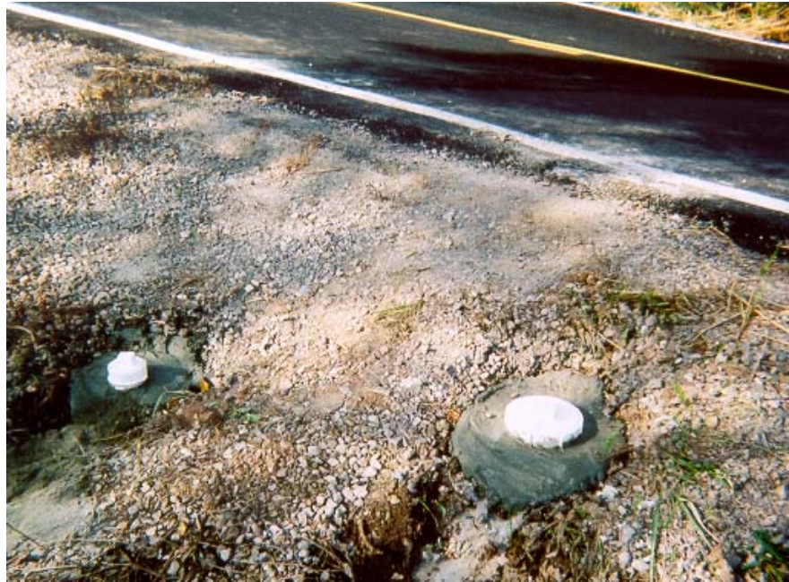
Figure 3.13 - Completed Installation of Inclinometer and TDR Cable
