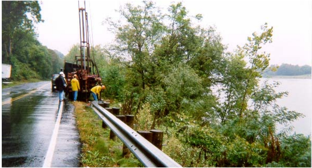
Figure 3.4 - Installation of Instrumentation at MEG-338 Site
