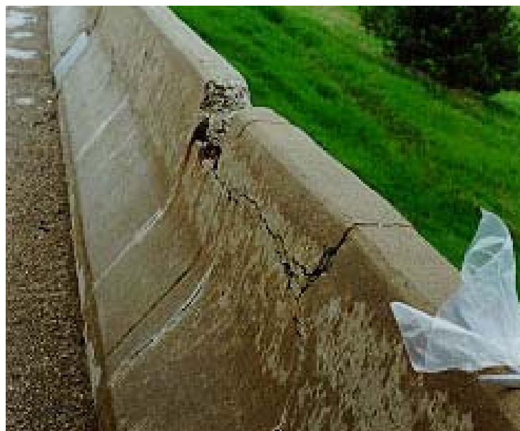
Figure 18A and 18B: Typical advanced deterioration of horizontal crack. Note the oxidation staining from the black reinforcing steel, further leading to expansion and ultimate failure of the concrete due to corrosion expansion.
