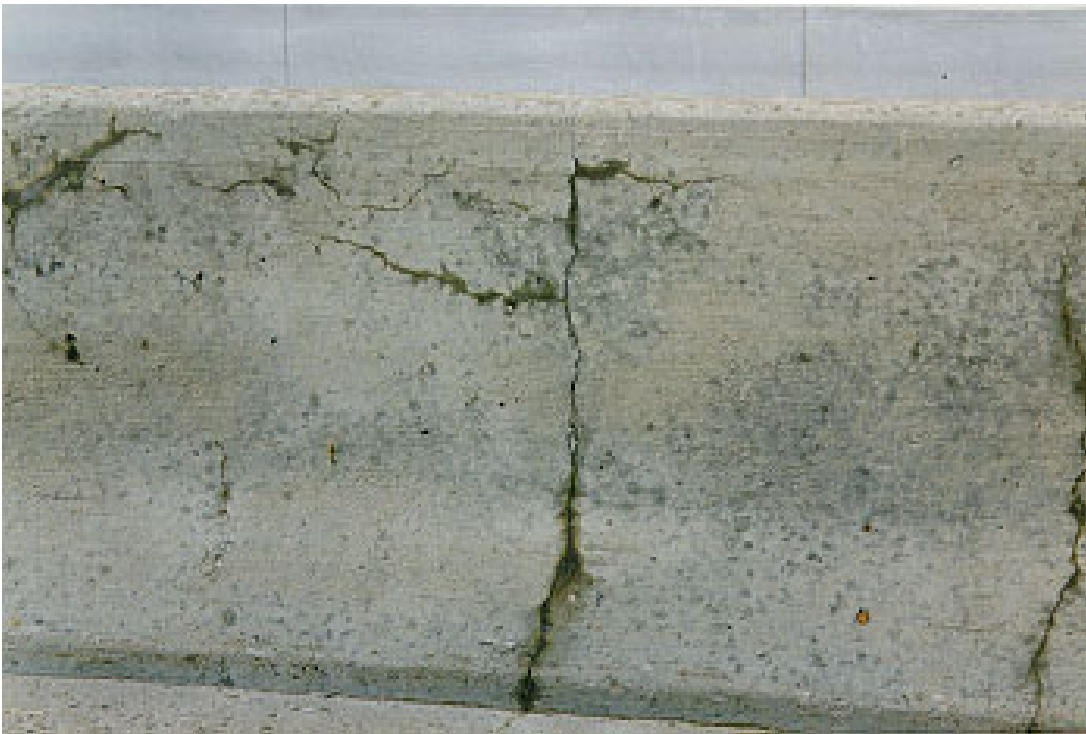
Figures 17A and 17B: S01 of 19042, EB I-69 over US-127 near Lansing, MI. Constructed in 1985, this slipform concrete barrier was constructed at the same time, using the same materials as the cast-in-place barrier described in Figure 16. The type and magnitude of distress is typical of slipform barriers in Michigan.
