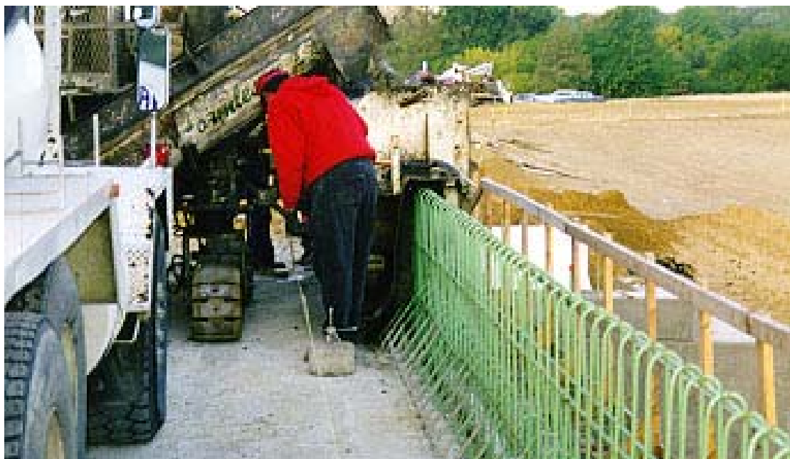
Figures 8A and 8B: Typical "slipform" concrete barrier operation.
