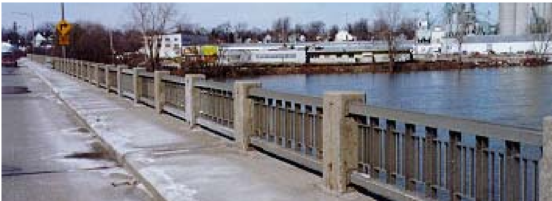
Figure 1A and 1B: Typical R-4 or R-5 standard bridge railing design prior to 1960.
