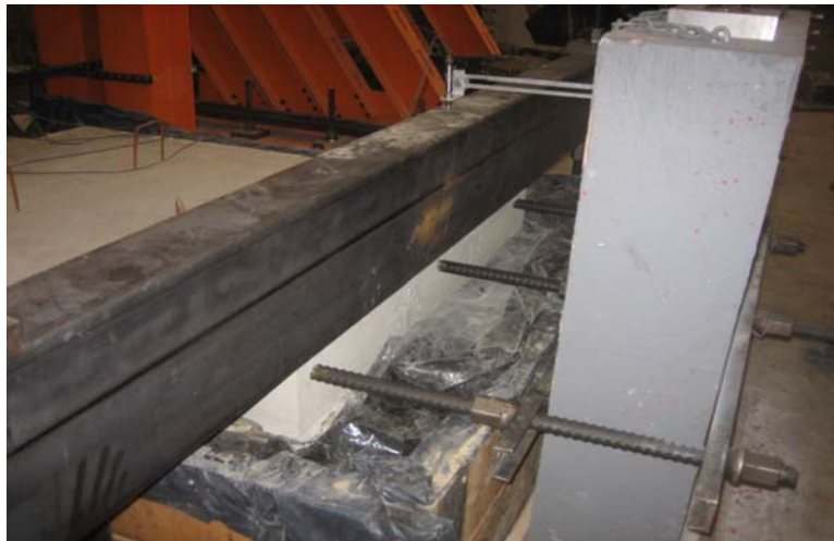
Figure 4.26 Threaded Rods Forced Against the Ends of the Slab
