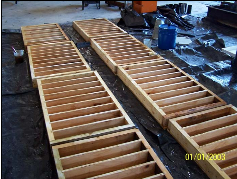
(a) The wooden formwork for casting 72 beams simultaneously
