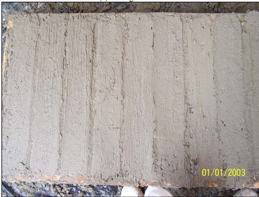
(b) Finished beams
