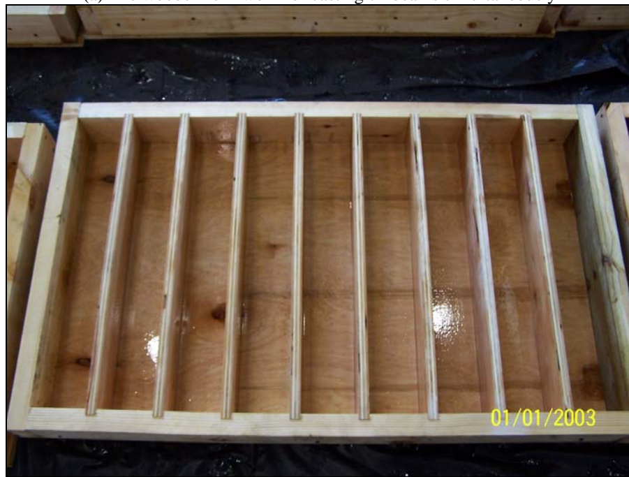
(b) Oiling of the formwork one day before pouring concrete
