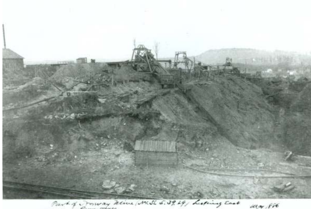
Figure 9 Photograph of an old iron mine showing the head frame at the top of the open pit.
