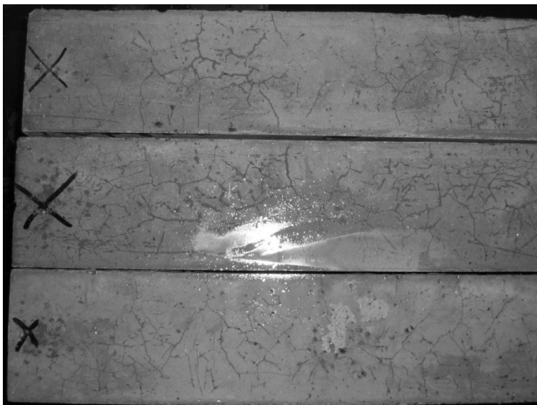
Figure 4-13: Cracks in Air Cured UHPC Specimens Following Freeze-Thaw Testing
