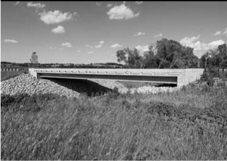
Figure 2-5: Mars Hill Bridge in Wapello County, Iowa (Lafarge 2006b)
