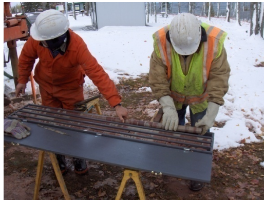
Figure 12: Rock cores being drilled and placed in boxes.
