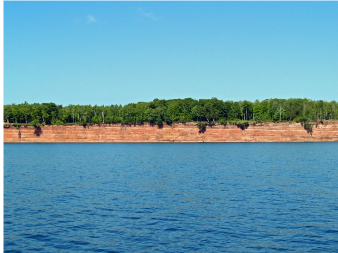
Figure 6: Section of consistent cliff structure north of MDOT Roadside Park; note the lack of talus slope formation due to direct long shore current removing the sandstone talus slope.
