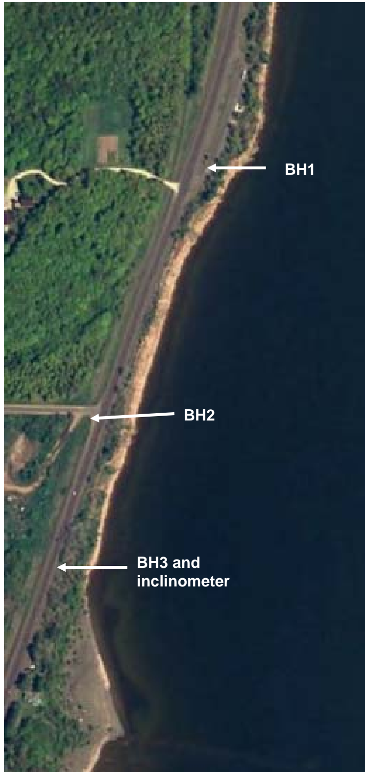
Figure 14: Approximate location of boreholes and inclinometer.
