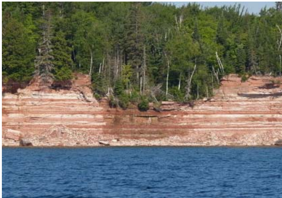
Figure 5: Seasonal stream causing accelerated erosion.
