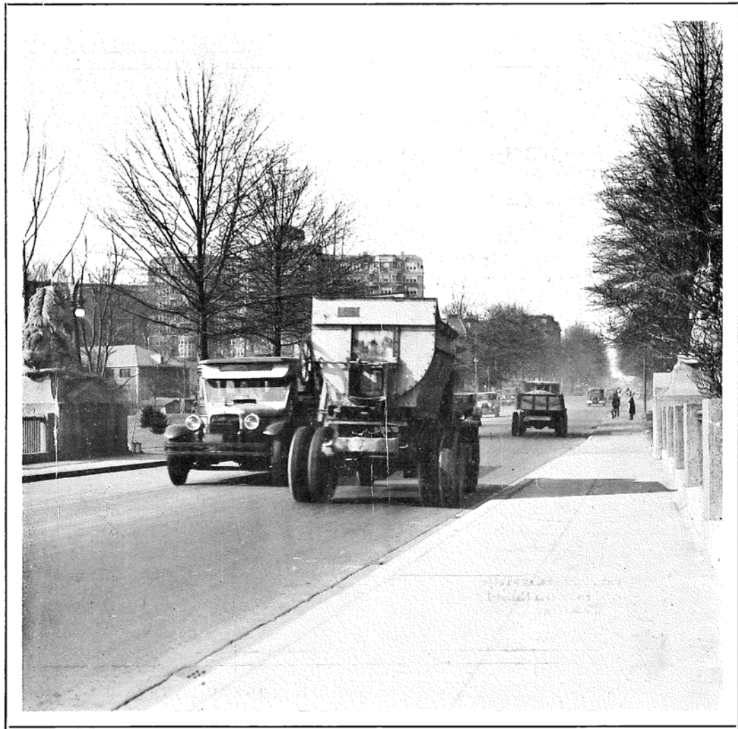
RESEARCH HAS RESULTED IN A BETTER UNDERSTANDING OF STRESSES IN CONCRETE BRIDGE SLABS
