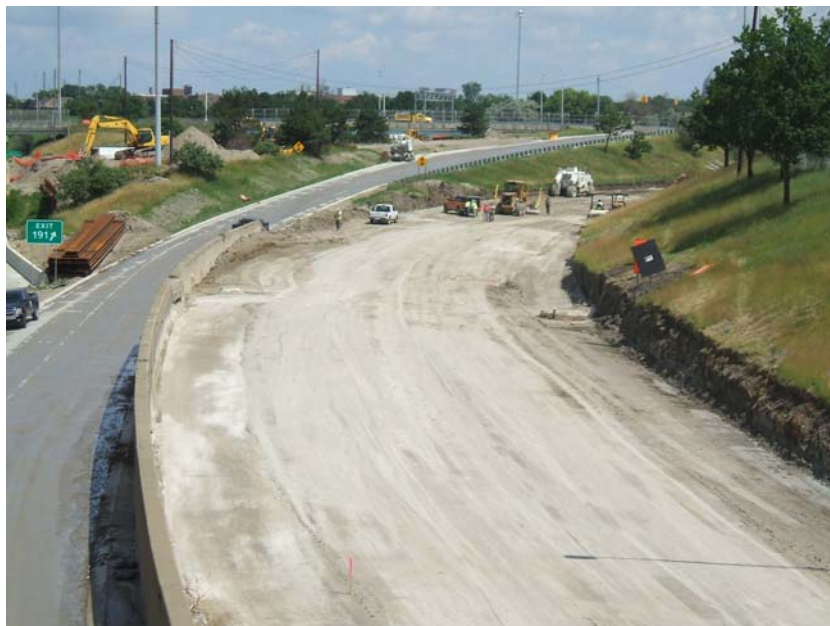
Figure 15: Finished Grade of Test Area 2
