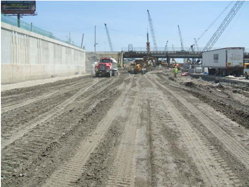
Figure 7: Grading
