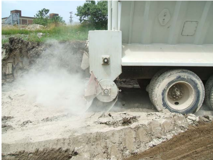
Figure 10: CKD Spreading on the Test Area 2
