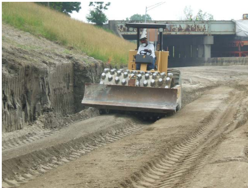
Figure 13: Rolling with Sheep Foot Roller
