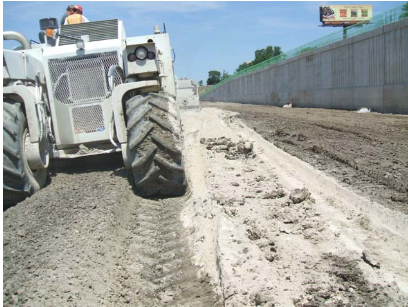
Figure 3: CKD Mixing with Rotary Pulverizer
