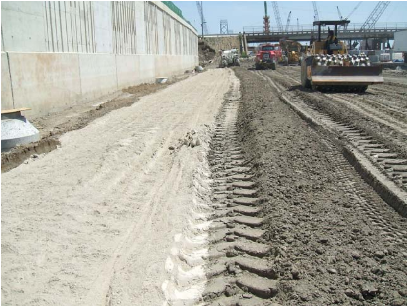
Figure 8: Finishing Different Areas of Test Area 1
