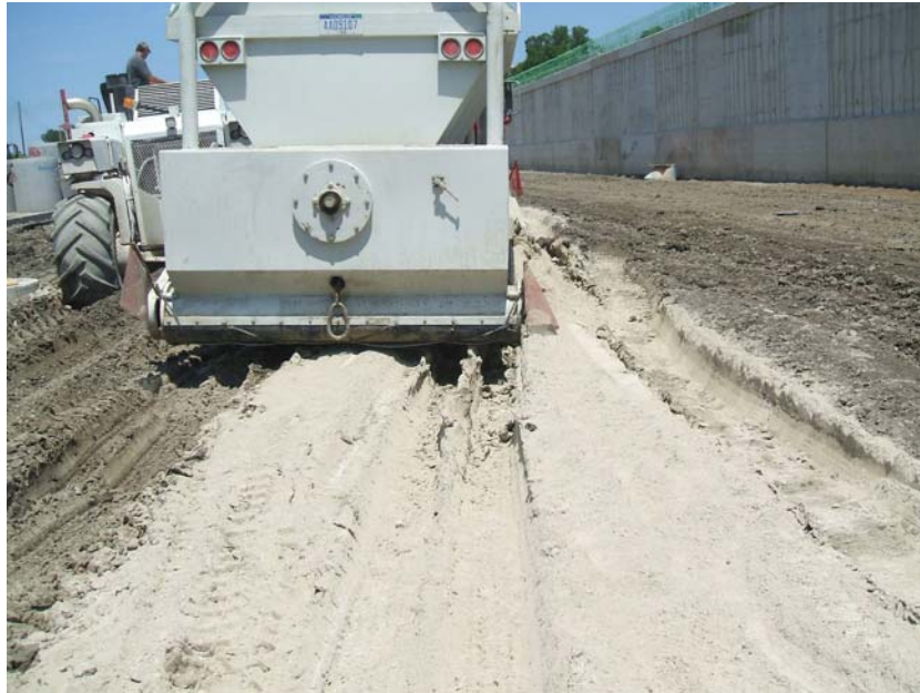
Figure 5: Spreader and Mixer working Side-By-Side
