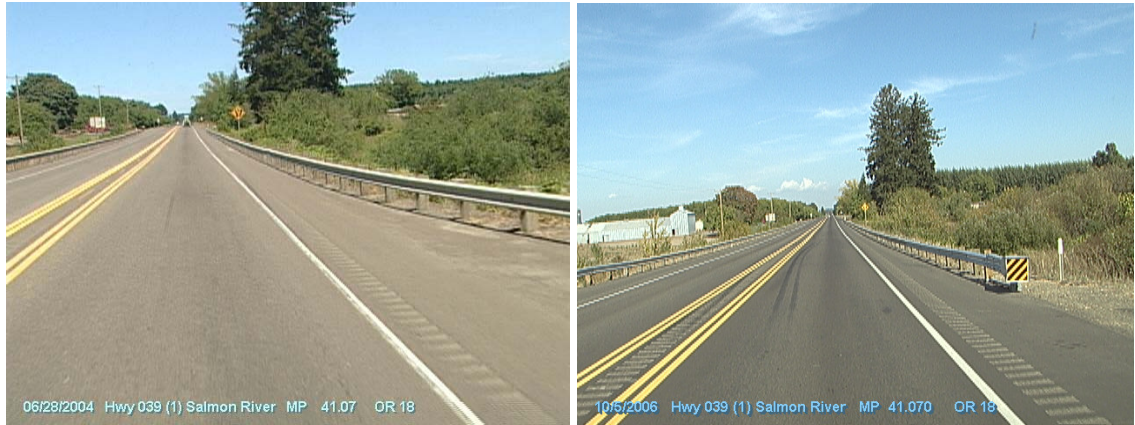
Figure 5.32: Conditions in 2004 (before) and in 2006 (after) showing the upgraded guardrail at MP 41.07
