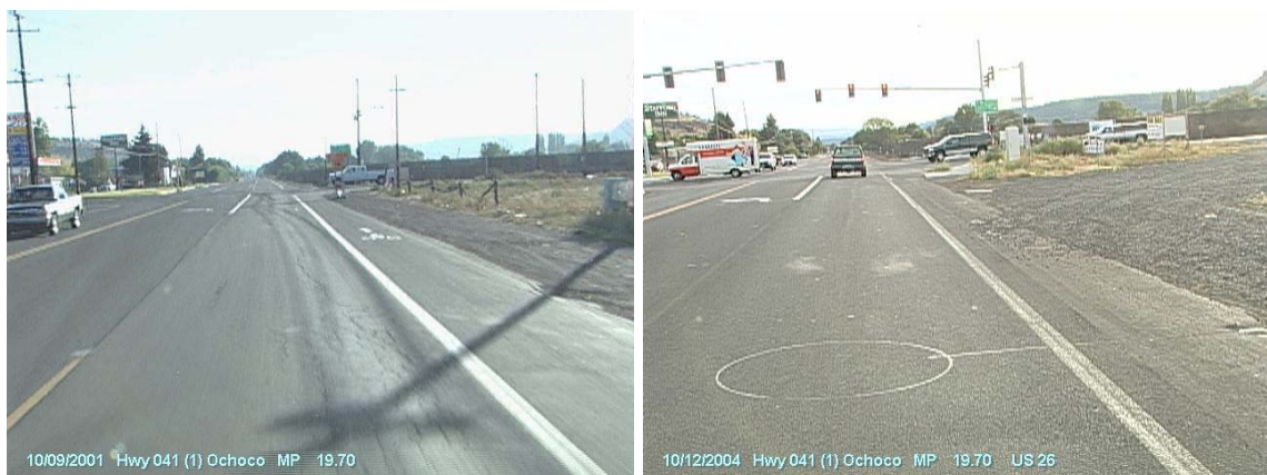
Figure 5.27: Conditions in 2001 (before) and in 2004 (after) showing the traffic signal installation at OR 126 and Combs Flat (MP 19.75)
