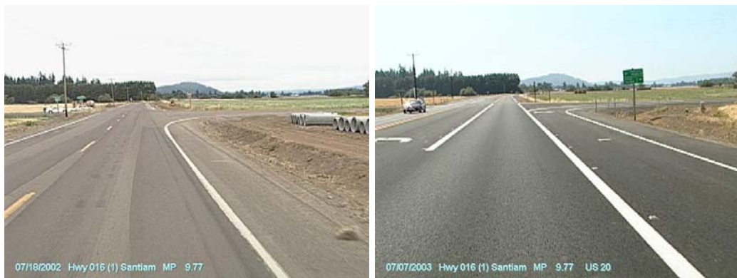
Figure 5.2: Conditions at Spicer Rd in 2002 (before) and added turn lanes in 2003 (after)
