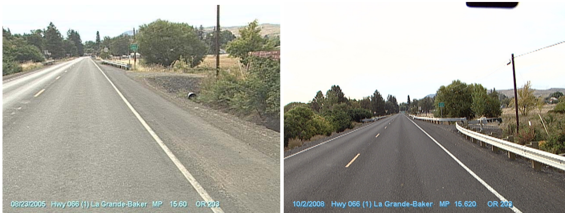
Figure 5.46: Conditions in 2005 (before) and in 2008 (after) showing the upgraded and new guardrail at MP 15.60
