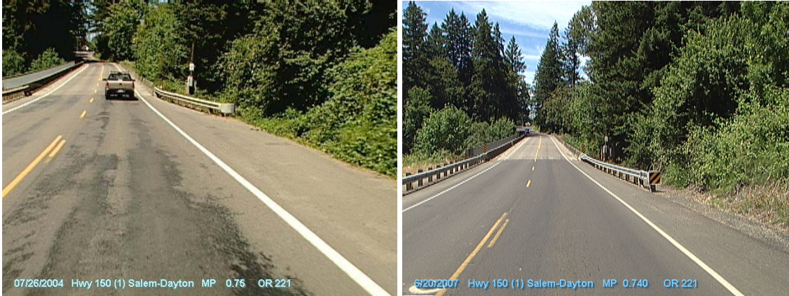
Figure 5.44: Conditions in 2004 (before) and in 2007 (after) showing the upgraded guardrail ends at MP 0.75
