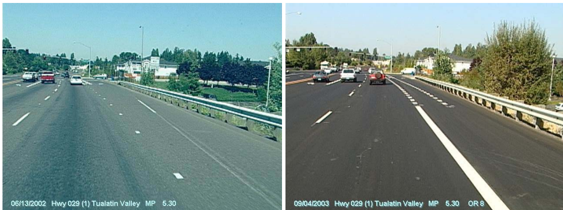
Figure 5.17: Conditions in 2002 (before) and in 2003 (after) showing the preservation work at MP 5.30
