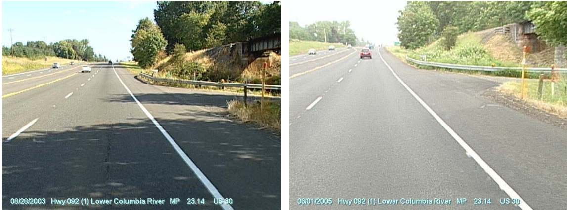
Figure 5.34: Conditions in 2003 (before) and in 2005 (after) showing the preservation work at MP 23.14
