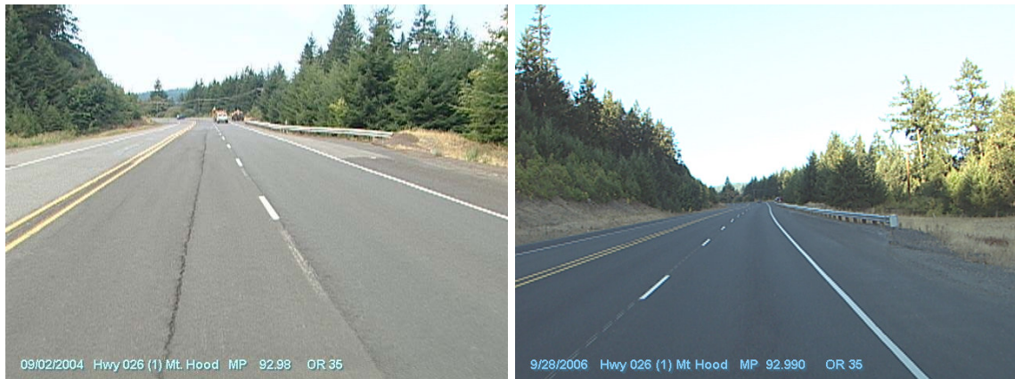
Figure 5.38: Conditions in 2004 (before) and in 2006 (after) showing upgraded guardrail at MP 92.98
