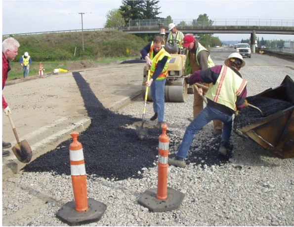
a) Covering gages with HMA.
