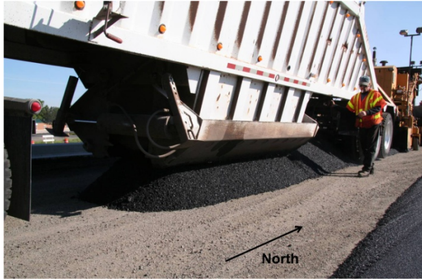
a) HMA windrow placed directly over partially protected gages.
