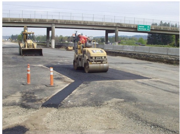
d) Compacting HMA with a small roller.
