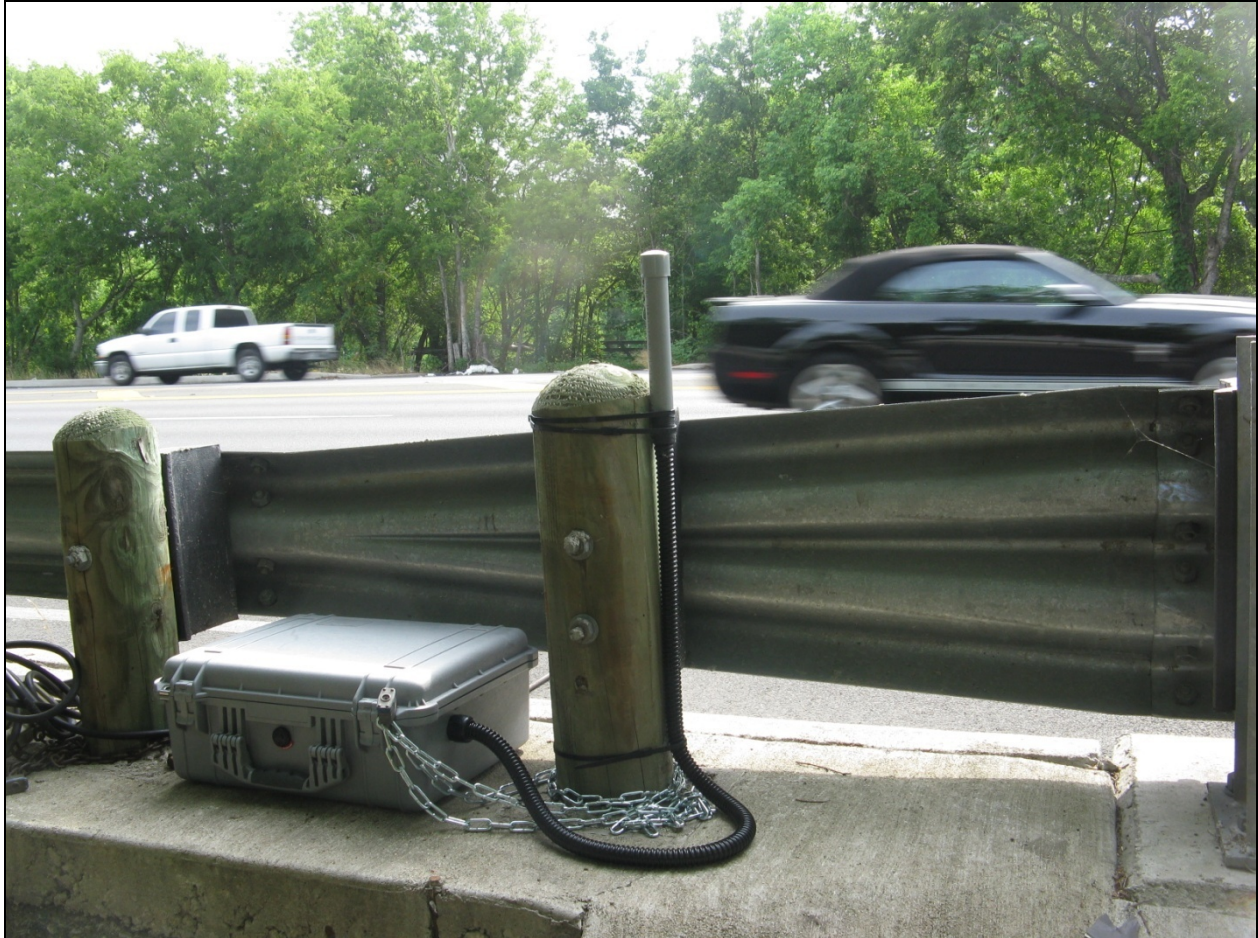
Figure 14. Highway 6 Portable Deployment
