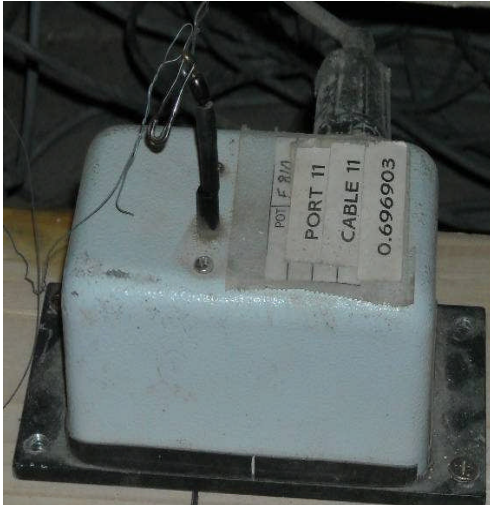
Figure 2.13 String Gauge Deflection Measurement
