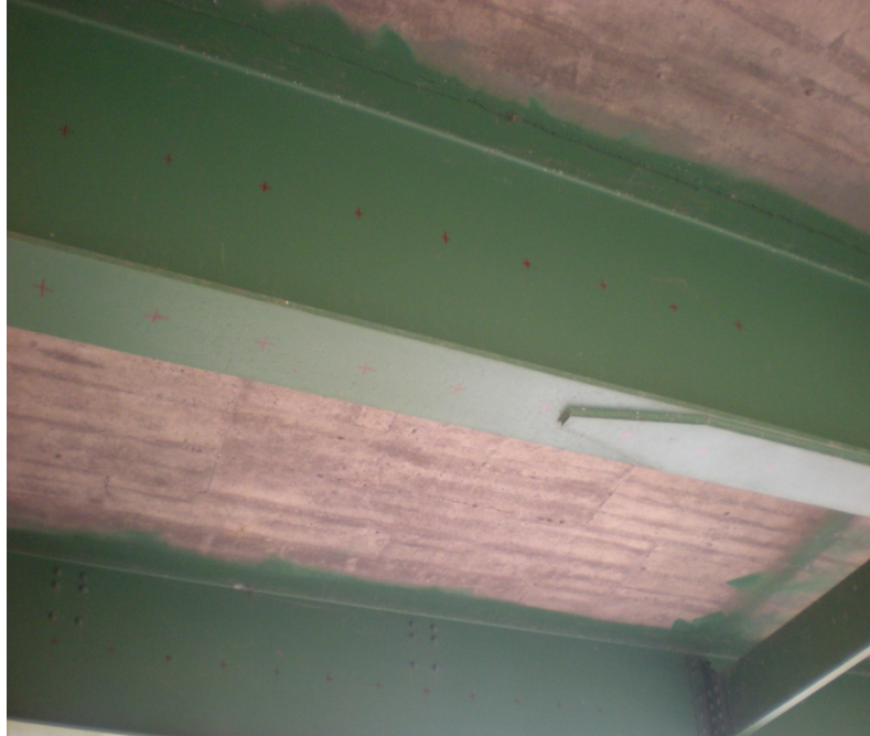
Figure 4.4 Markings at one foot intervals on the web and bottom flange of each beam
