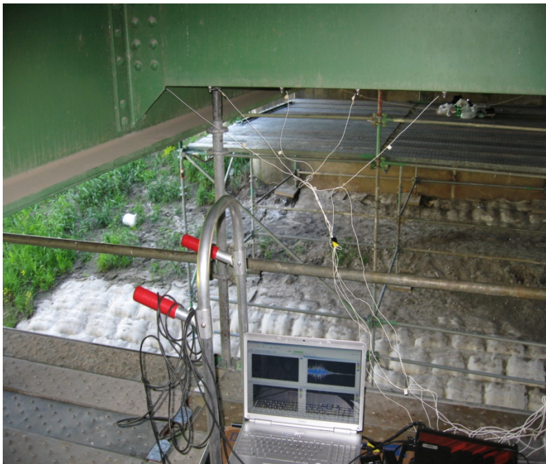
Figure 4.26 Operational vibration response measurement of a diaphragm member
