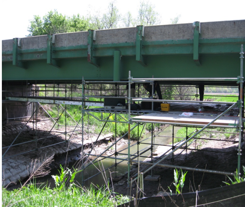
Figure 4.13 Scaffolding that provided access to the entire superstructure
