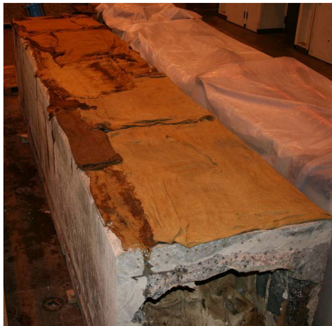
Figure 6-4: Burlap Soaking the Bottom of the Beam
