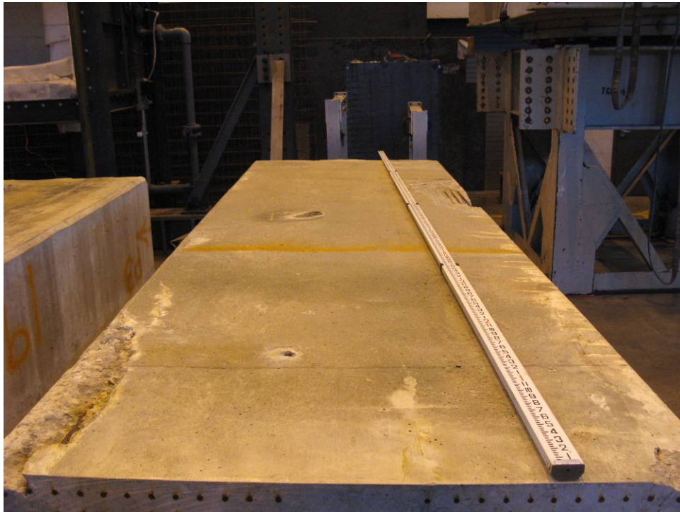
Lakeview, Beam 16, Span 2, Looking Ahead
