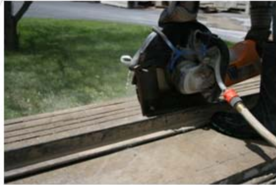
(b) electric concrete saw
