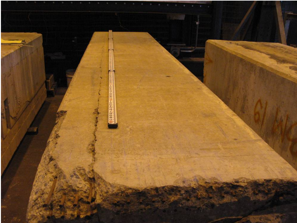
Clearfield, Beam 4, Span 2 , Looking Back
