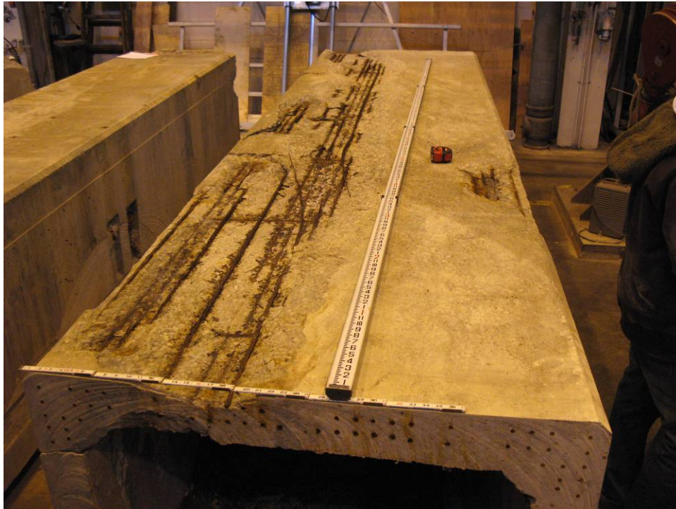
Main Street, Beam 2, Span 3, Looking Ahead
