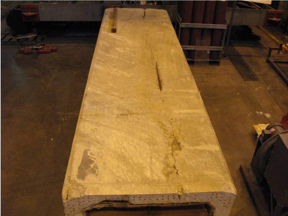
Main Street, Beam 3, Span 3, Looking Ahead
