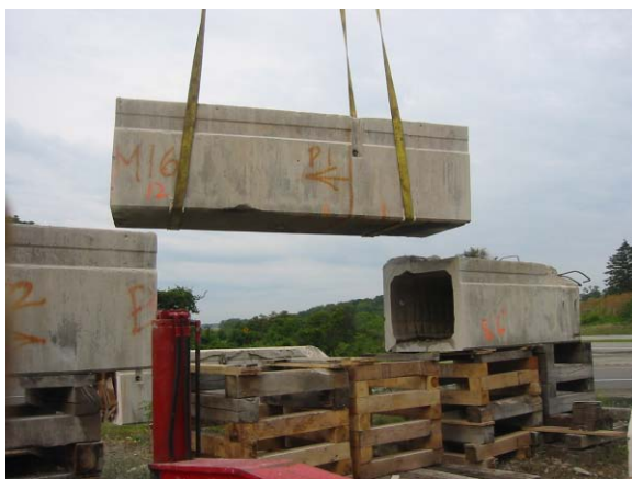
c) Field Handling of Cut Sections
