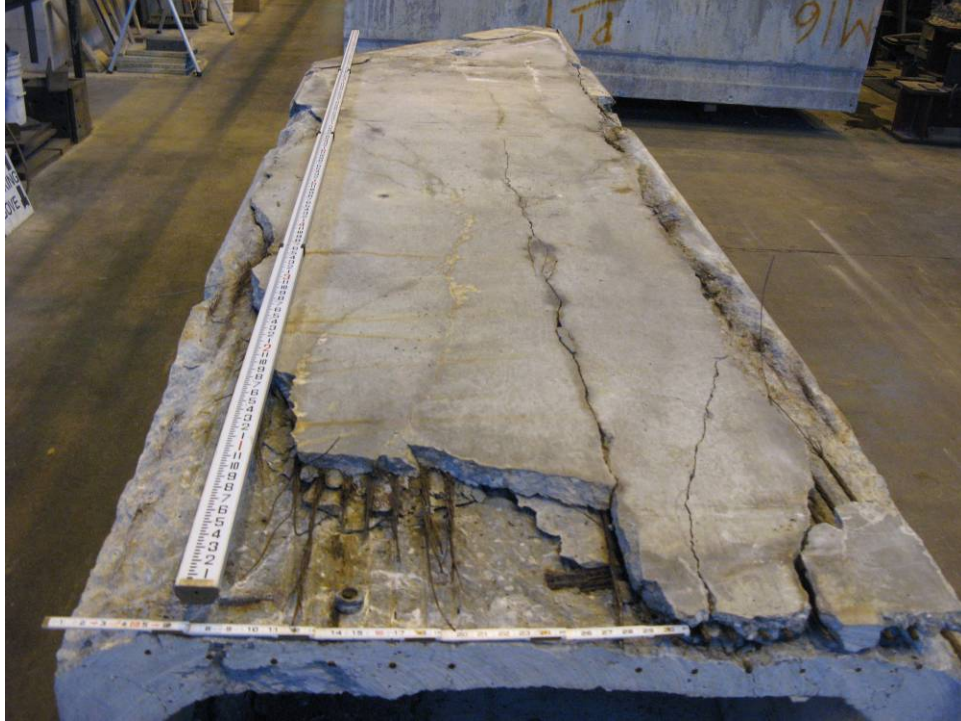
Lakeview, Beam 7, Span 1, Looking Back
