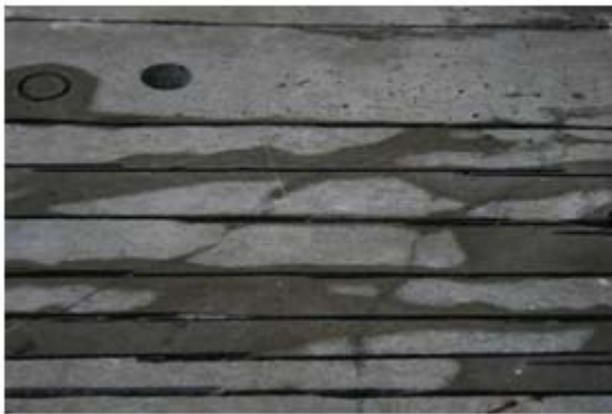
(a) After Cutting
