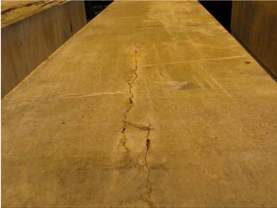
Clearfield, Beam 3, Span 1, Looking Ahead
