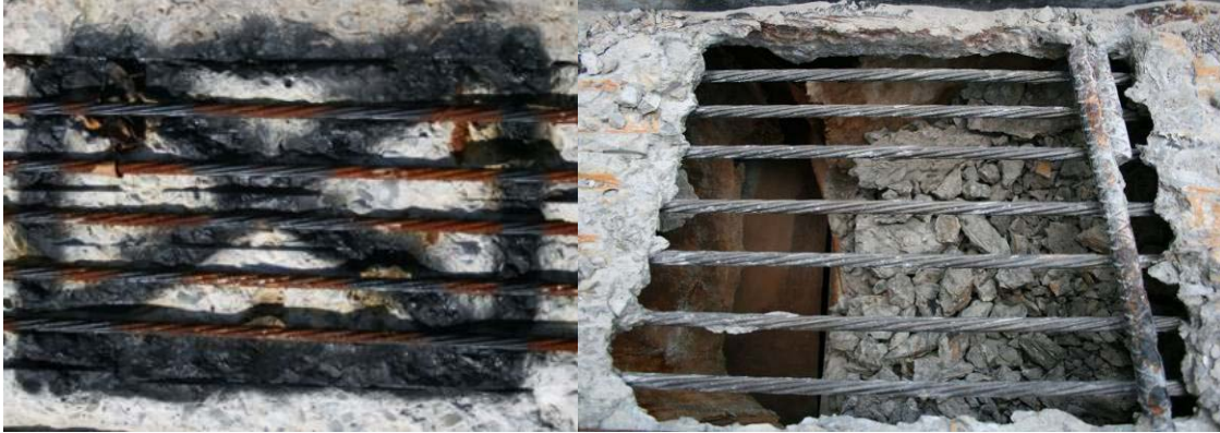
Figure 5-10: Before and After Deconstruction
