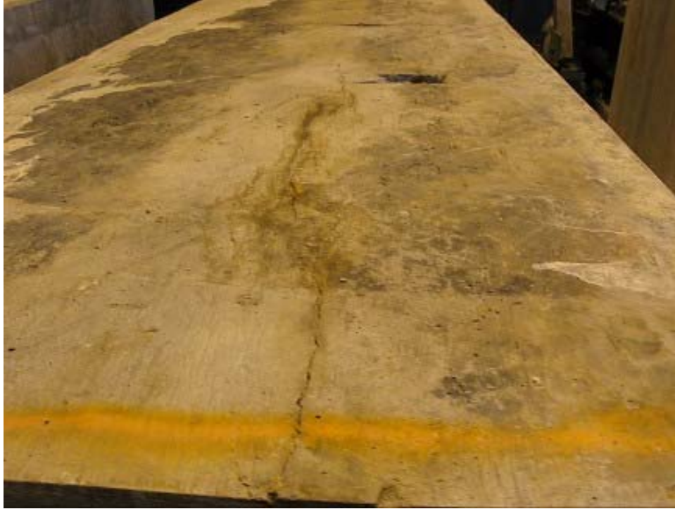
Lakeview, Beam 19, Span 3, Looking Ahead
