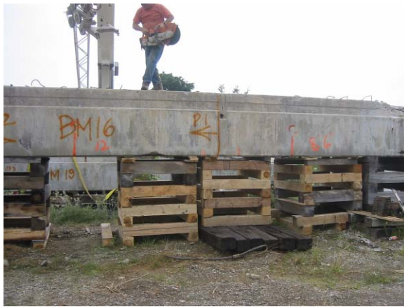
a) Beam Support and Staging
