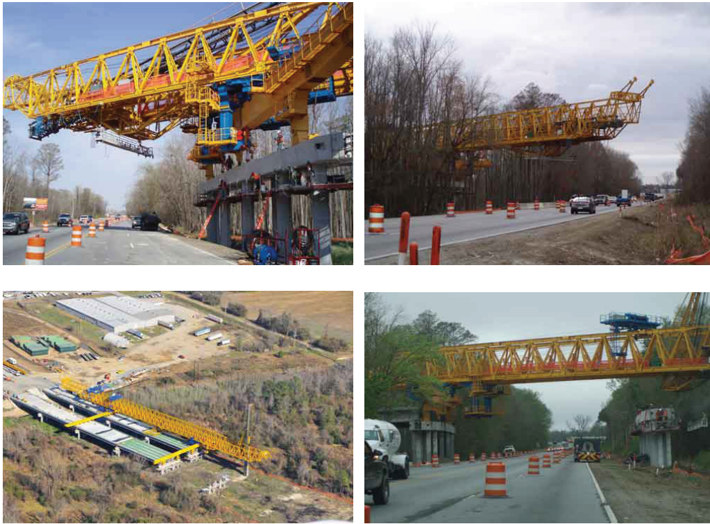
FIGURE 5: NORTH CAROLINA WASHINGTON BYPASS BRIDGE: DESIGN-BUILD INNOVATION
