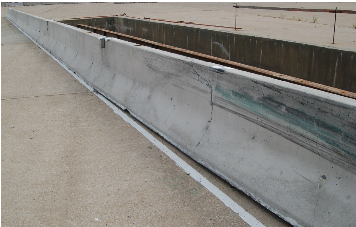
Figure 26. System Damage, Test No. NYTCB-5
