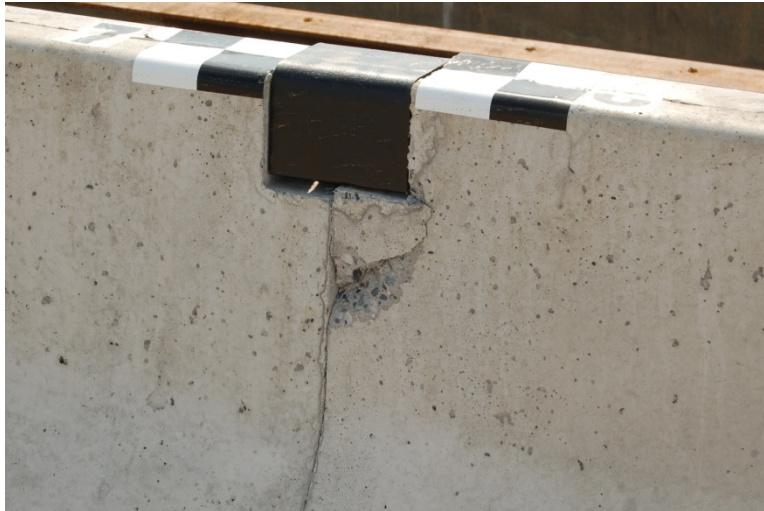
Joint between Barrier Nos. 6 and 7
