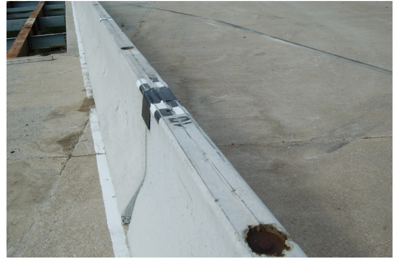
Joint between Barrier Nos. 9 and 10
