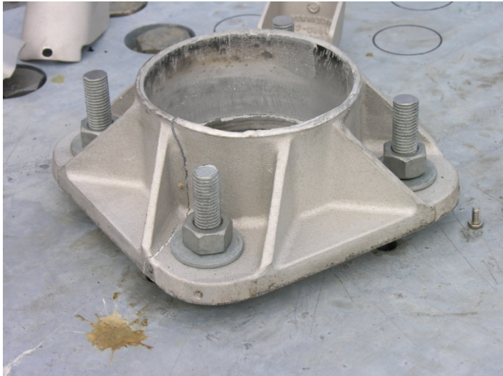
Figure 34. System Damage - Base Plate Cracks and Fractures, Test No. NYPP-1
