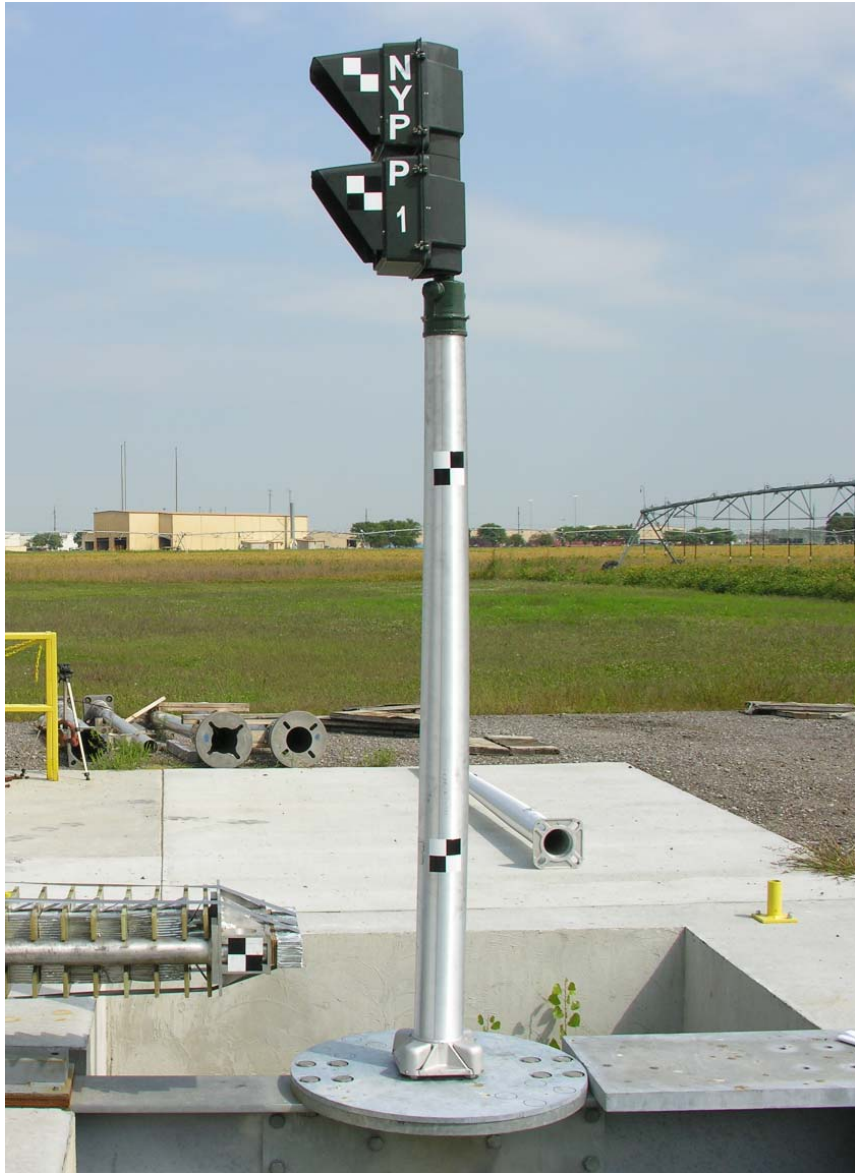
Figure 27. Assembled Pedestrian Signal Test Installation
