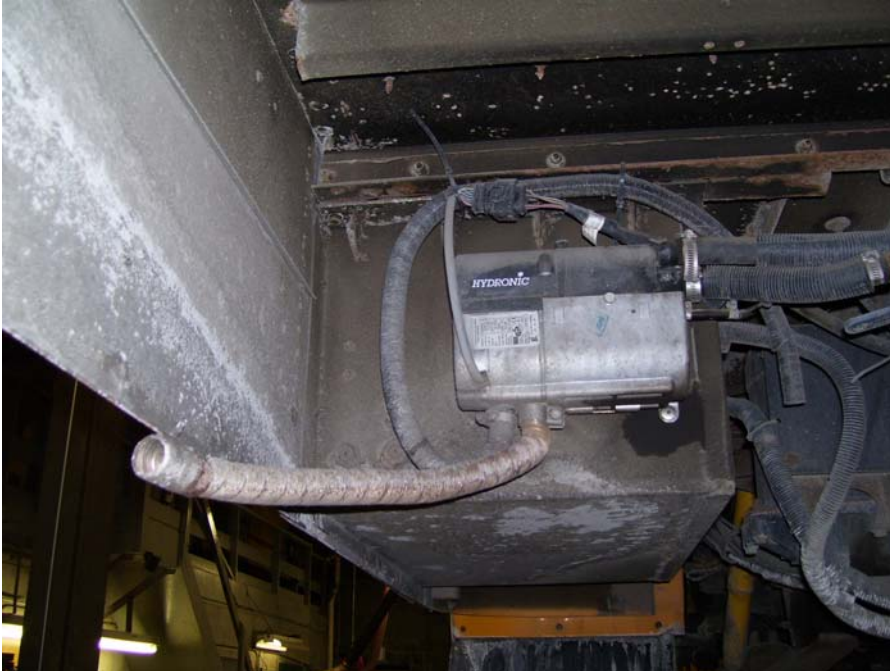
Figure 2 - Espar Auxiliary Heater Installation
