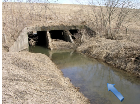
Considerable clogging appears on the right and central boxes of the culvert. The left box is clean; the others are heavily sedimented (about 1 m elevation difference).
