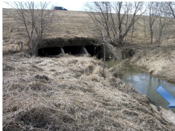
Considerable clogging appears on the right and central boxes of the culvert. The left box is clean; the others are heavily sedimented (about 1 m elevation difference).
