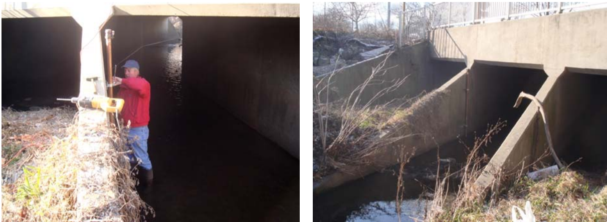
Figure 3-11 Setup of the water level sensor: a) during the installation of the sensor; b) the sensor in its working position
