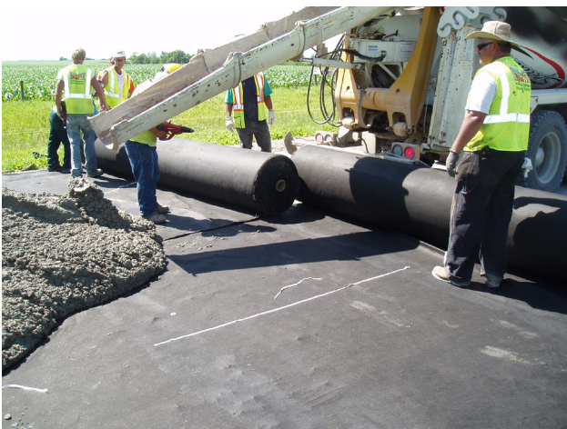
Installing geotextile material as an innovative bond breaker in Poweshiek County
