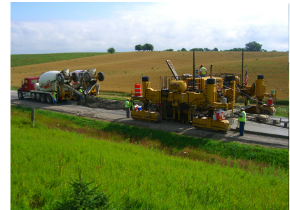
Two-lane stringless paving in Poweshiek County
