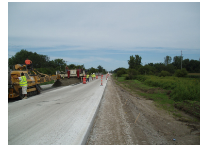
Single-lane paving with stringline in Johnson County
