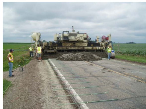
Figure 12. Dual Lane Paving with a Stringline Requires Complete Road Closure
