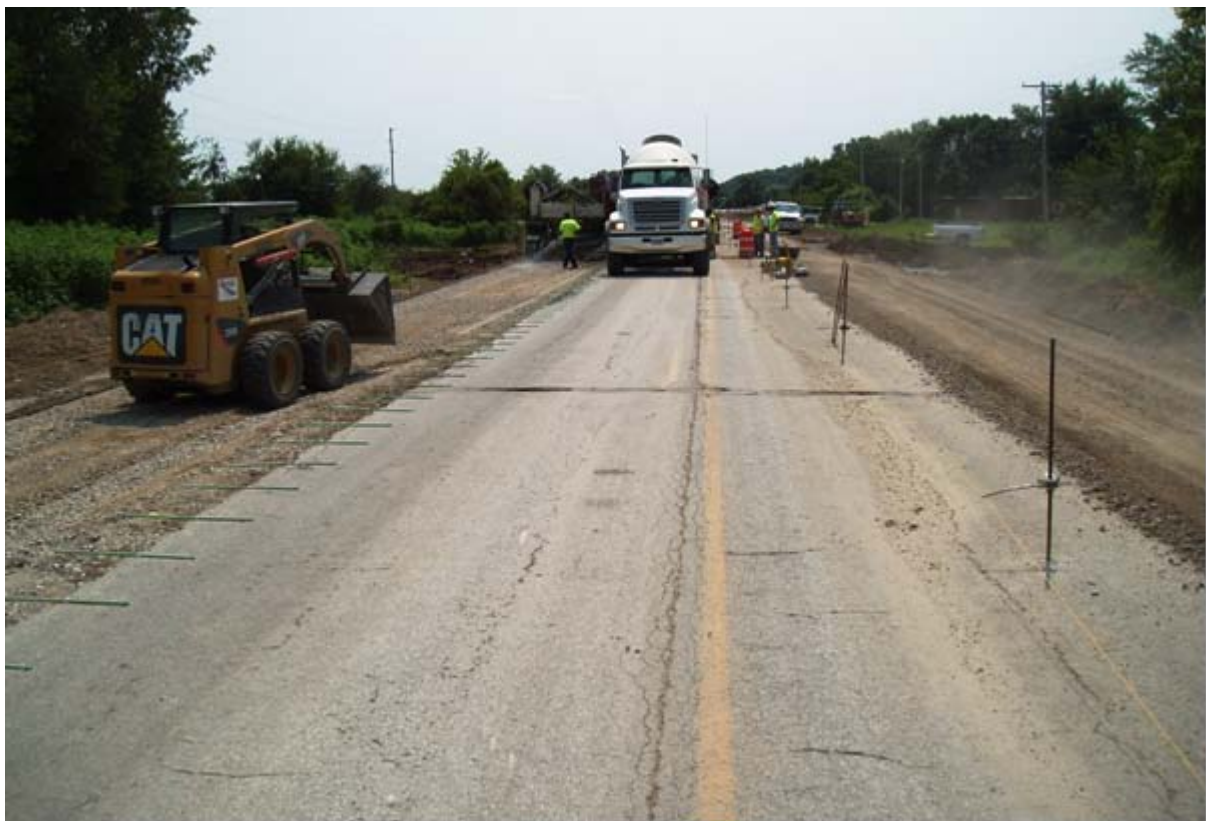
Figure 10. Construction on W-62 in Johnson County while maintaining local traffic
