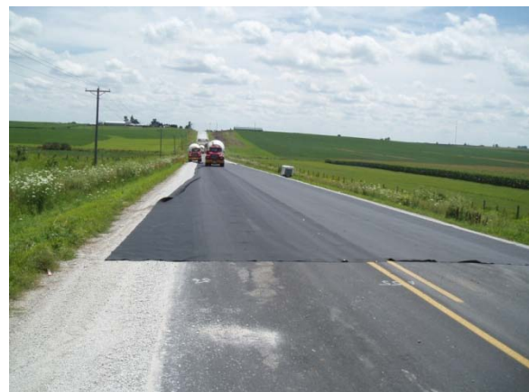
Figure 9. Equipment Operating over Geotextile Bond Breaker
