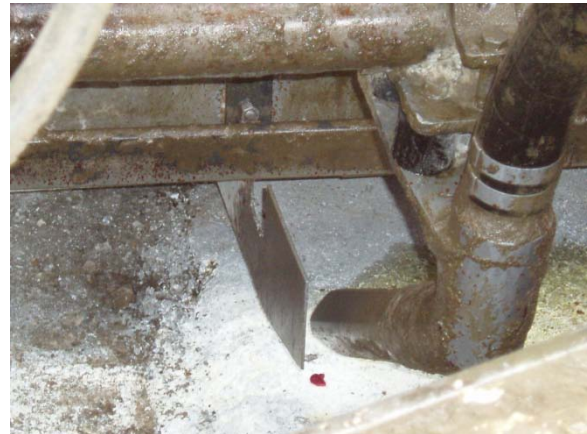
Figure 14. Longitudinal Joint “Knife” Installed on Slipform Paver
