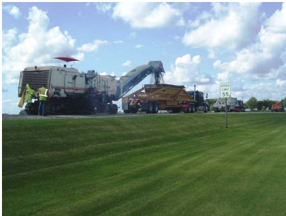
Figure 6. Mainline Pavement Milling
