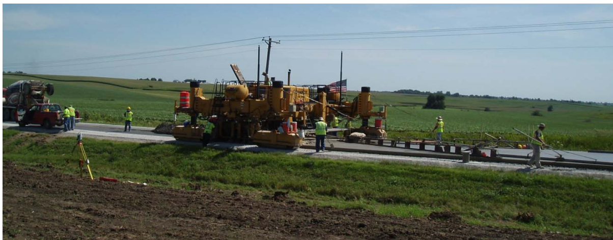
Figure 3. Dual Lane Stringless Paving Operation
