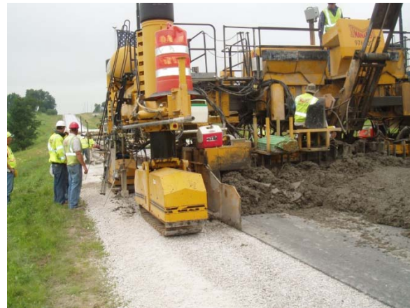
Figure 2. Slipform Paver Utilizing Stringless Paving
