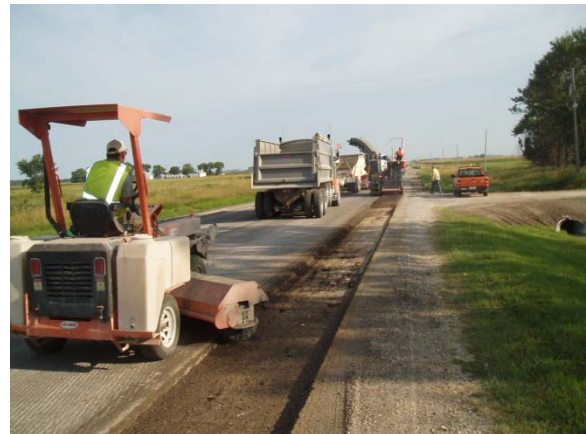
Figure 7. Shoulder Milling for Pavement Widening
