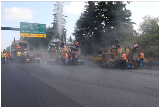
Figure 12. At times, three paving machines and two Shuttle Buggies were used.
