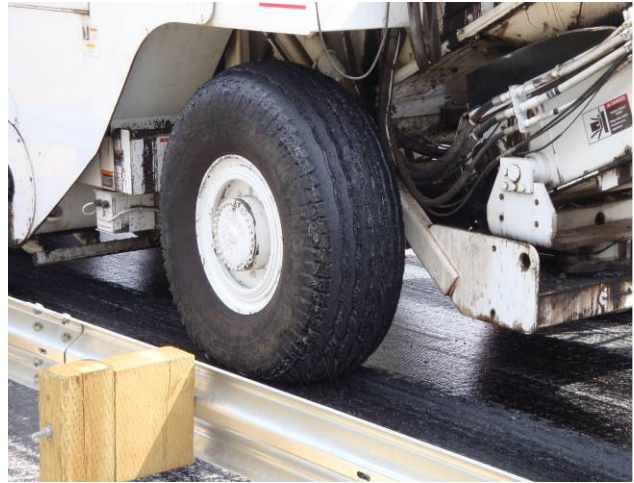
Pickup of tack when temperature was warmer
