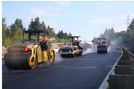
Figure 13. Rollers stayed close behind the paving machines.
