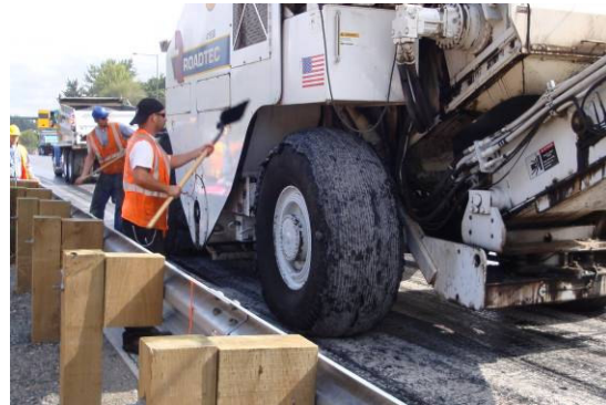
Figure 19. Members of paving crew removing tack buildup.
