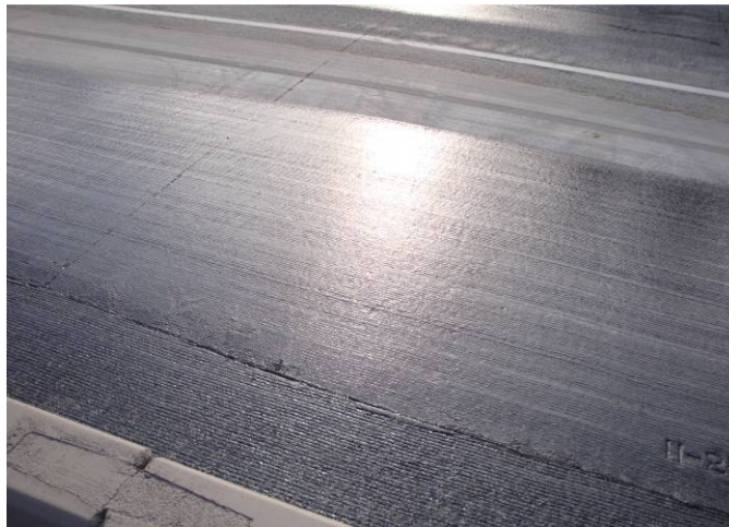
Image of tack application on new PCCP surface
