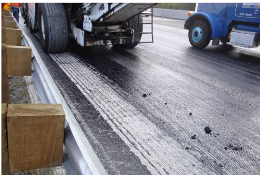
Figure 16. PG asphalt tack coat sticking to Shuttle Buggy tire in HOV lane.
