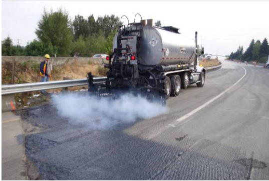
Figure 8. Distributor applying tack coat.
