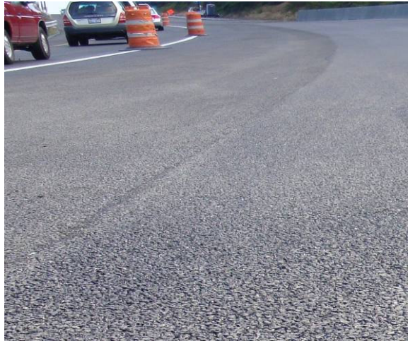
Image of the longitudinal joint
