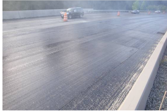
Figure 9. Tack coat application.
