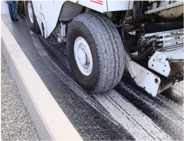
Image of tack pickup on new PCCP
