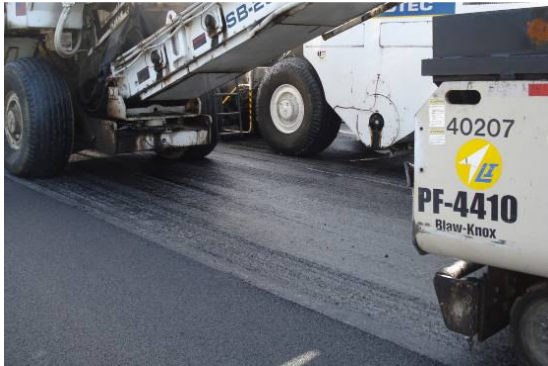
Figure 18. PG asphalt tack coat sticking to tires was not a problem on the old PCCP.
