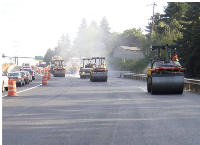
Looking at breakdown and intermediate rollers
