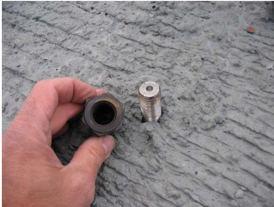
Figure 6 Typical elevation reference point
