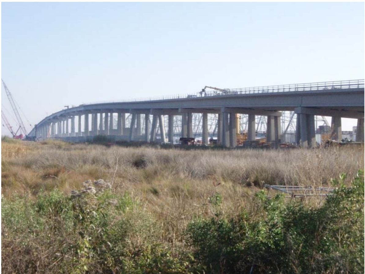
Figure 1 Rigolets Pass Bridge
