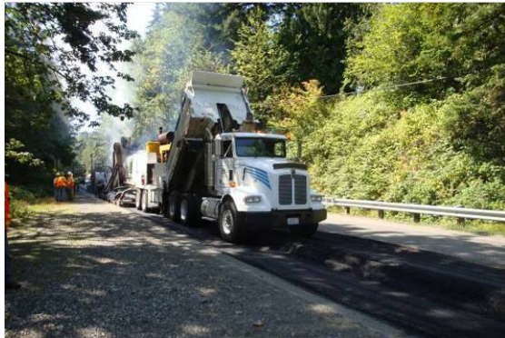
Figure 10. Truck dumping admixture into hopper of unit B.
