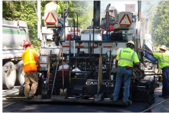
Figure 13. Rear view of RoadTec paving machine.
