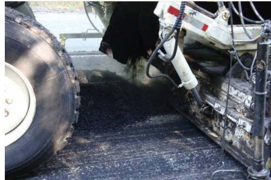
Figure 11. Millings from the full width milling head on unit B (right side of photo) are windrowed with millings from conveyer (top center).
