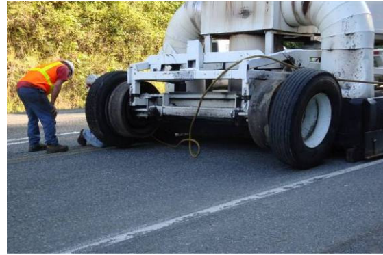
Figure 3. Removing rubber tires prior to paving.
