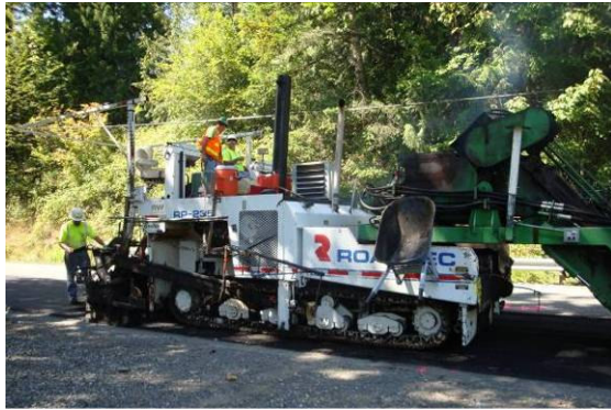
Figure 12. RoadTec RP 235 paving machine.
