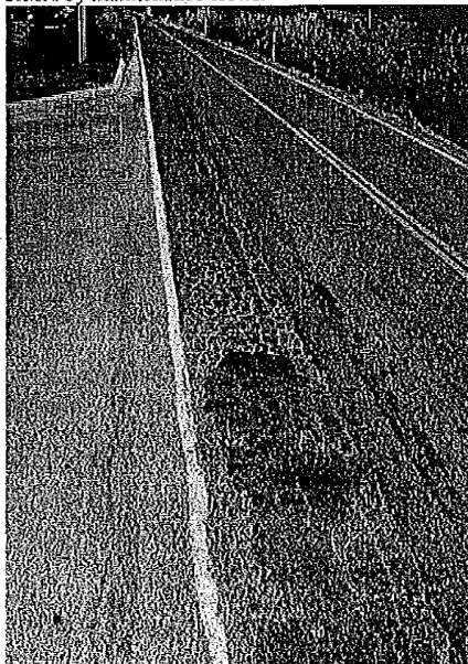
Photos 9 & 10 (SR 9 at ~ MP 84.06): Medium to high severity alligator cracking occurring in the wheel path between the edge of the PCCP panels and HMA pavement.
