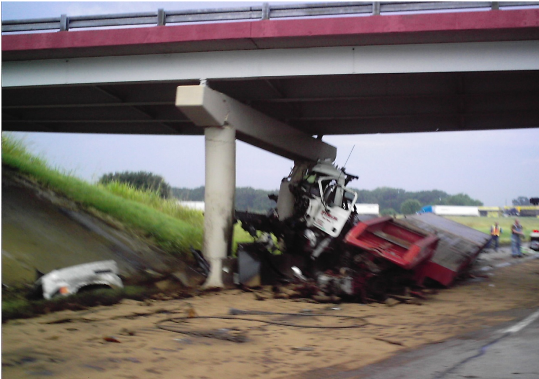
Figure 2.12. Truck Accident – Mile Post 519 Bridge over IH-20, Canton, Texas.
