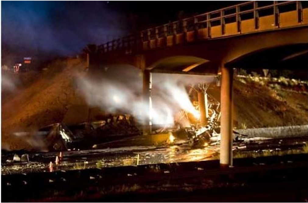
Figure 2.8. Truck Accident – Bridge on 26½ Road over IH-70, Grand Junction, Colorado.
