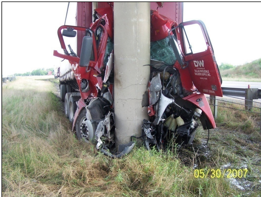
Figure 2.2. Truck Accident Chatfield Road Bridge, IH-45, Navarro County, Texas.
