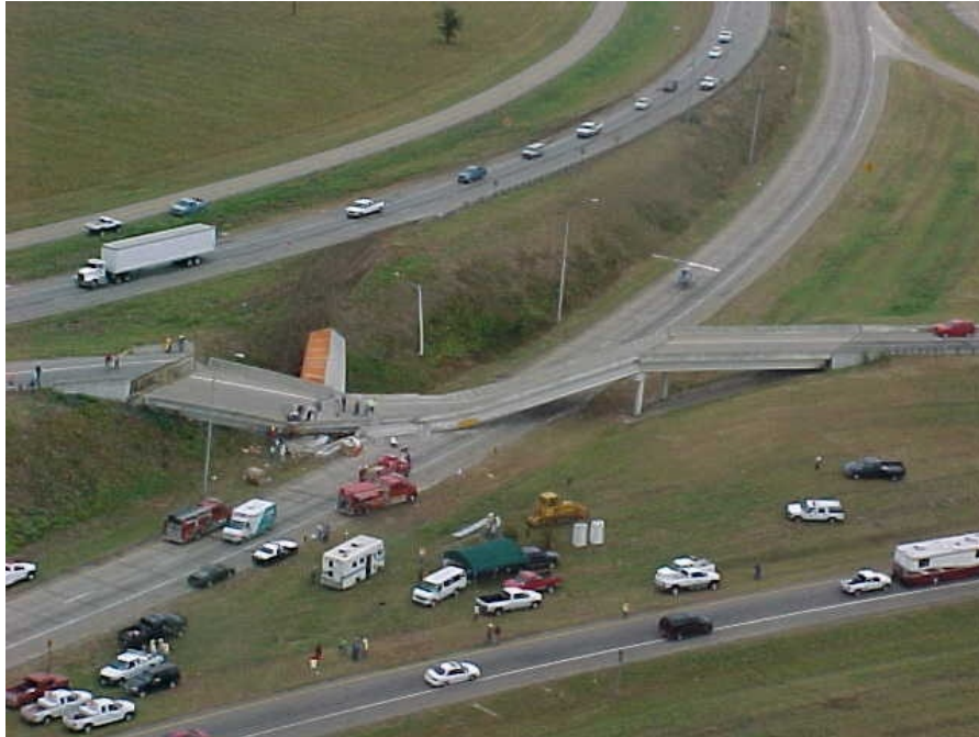
Figure 2.7. Truck Accident – SH 14 Bridge over IH-45, Corsicana, Texas.
