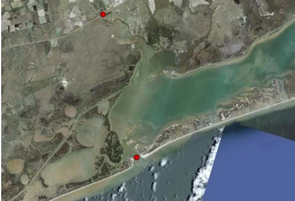
Figure 11. Bridges (Red Dots) of FM 2004 Road (Top Dot), and San Luis Pass (Bottom Dot) in Galveston. (Google Satellite Image, 2009e)
