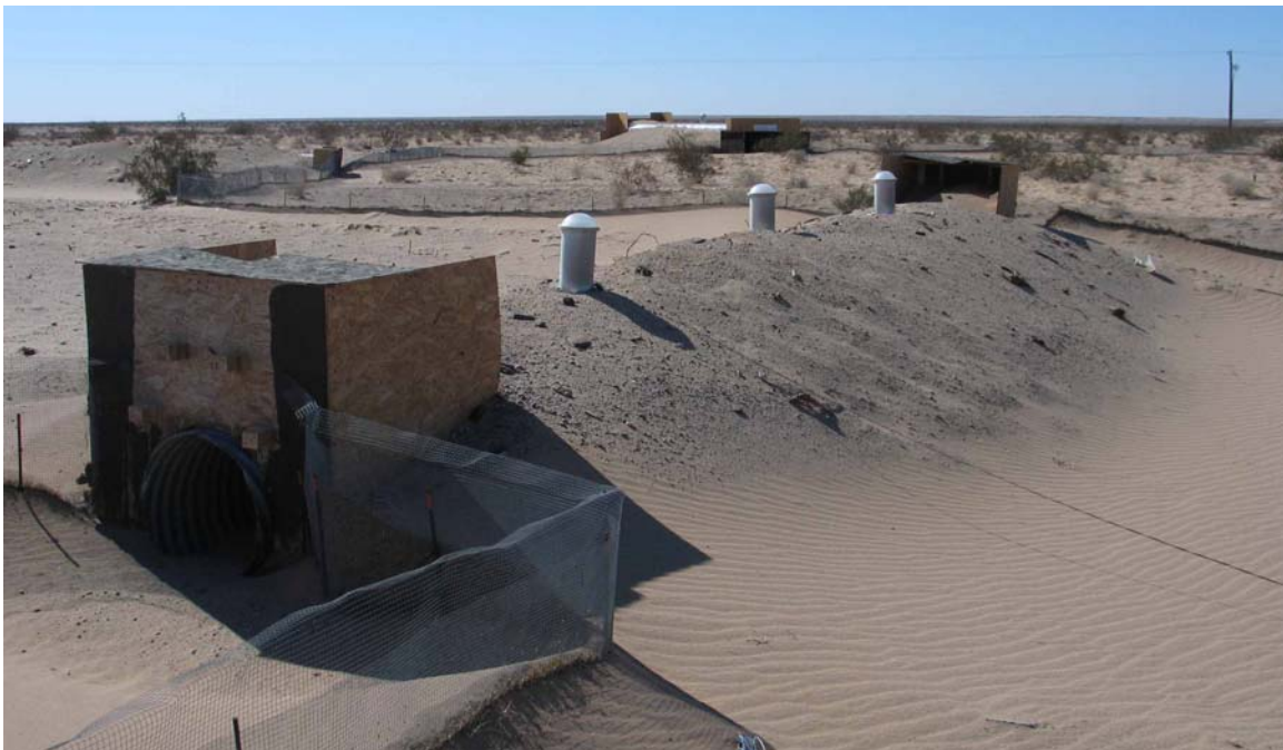
Figure 5. Skylights positioned on a 24-in diameter culvert.
