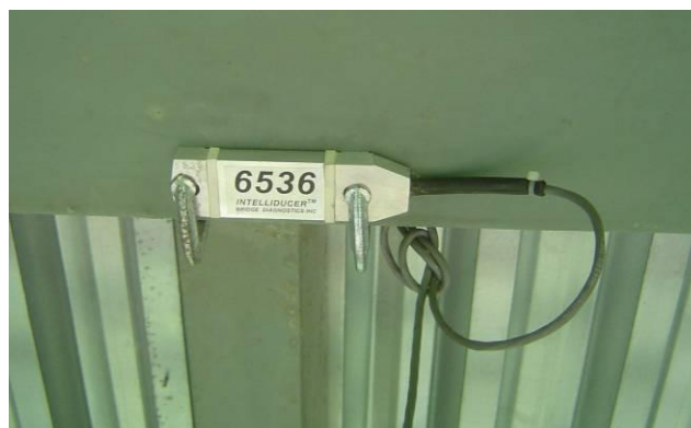
Figure 14. Strain transducer clamped to a stringer at the Pearl Harbor Memorial Bridge
