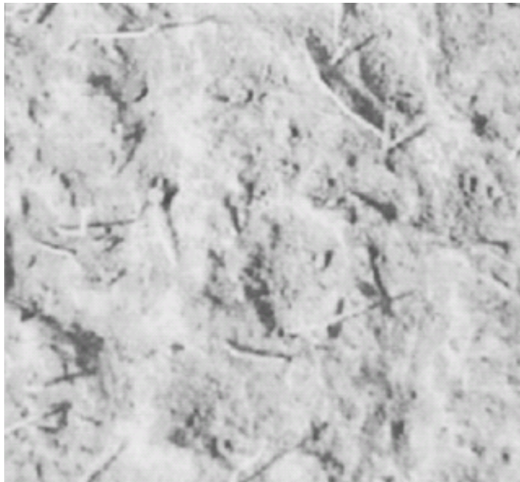
Figure 3. Separation of fiber on pavement surface ( Lin and Wang 2005 )
