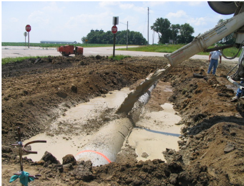
Figure 49. Pouring the flowable mortar
