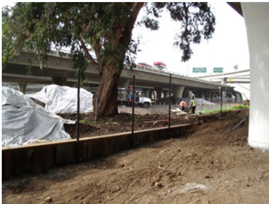
Figure 10 Emergency Preparedness: Building Trusses to Prevent Mudslides in Downtown San José
