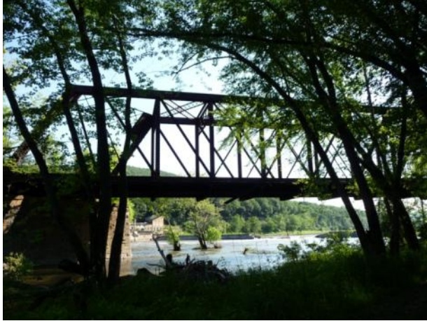
a) View from downstream (left side)
