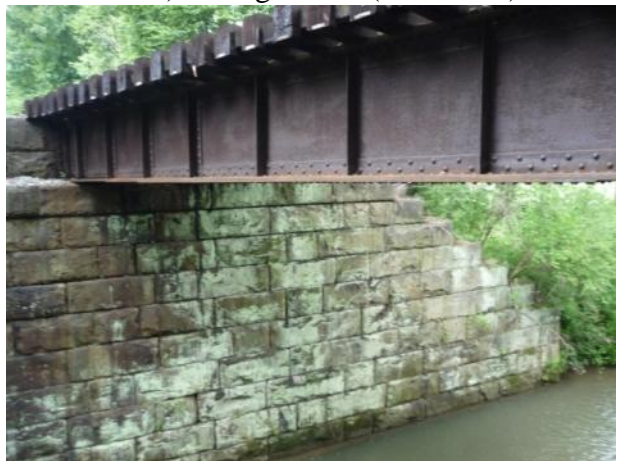
d) Plate Girder / Abutment
