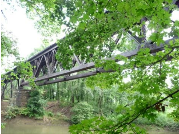
a) View from downstream (left side)
