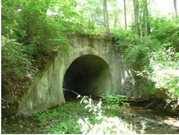
a) View from upstream (left side)
