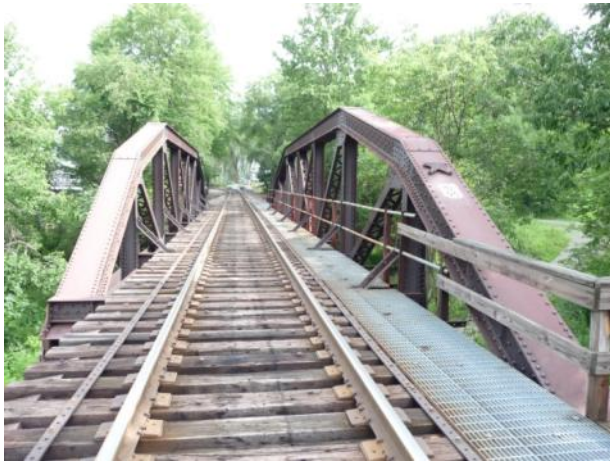
c) Bridge Approach (MP ahead)
