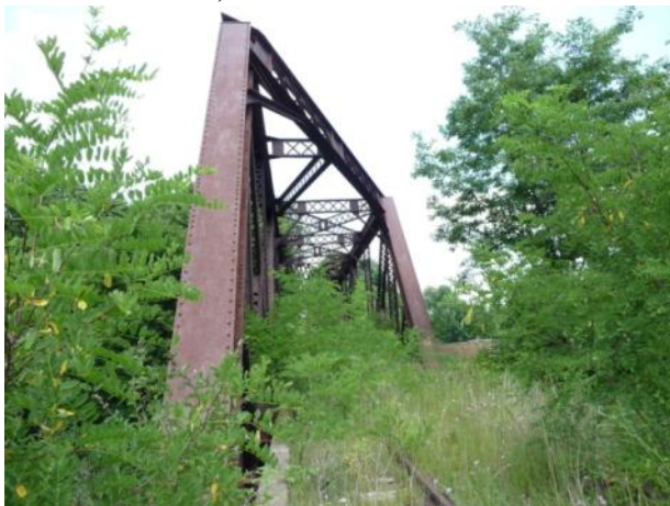
c) Bridge Approach (MP ahead)
