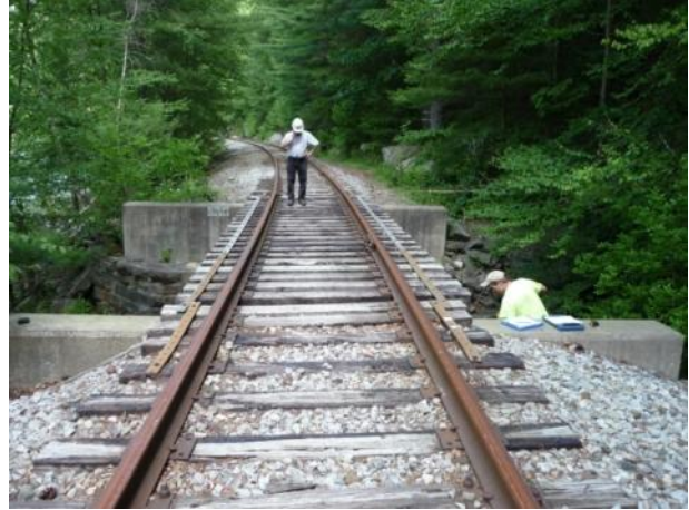
b) Bridge Deck (MP back)
