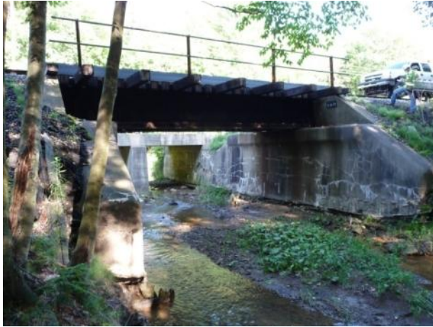
a) View from downstream (left side)
