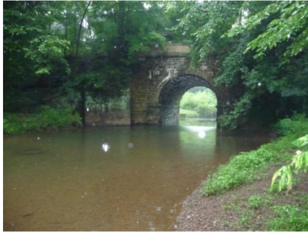
a) View from downstream (left side)
