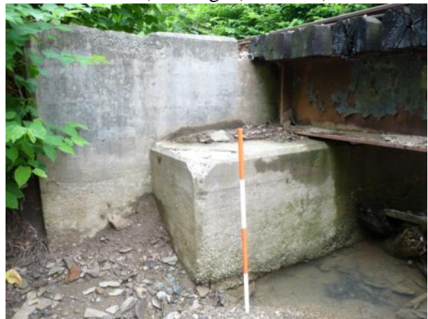
d) Abutment (near)
