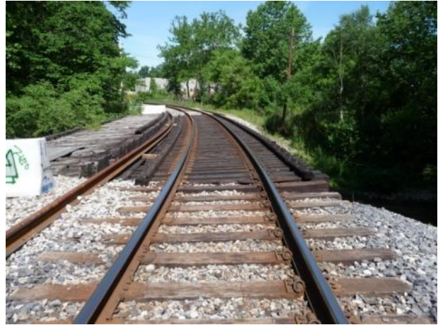
b) Bridge Deck (MP ahead)
