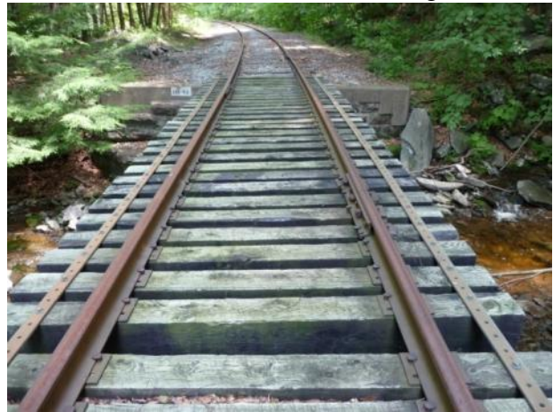
d) Bridge Deck (MP back)
