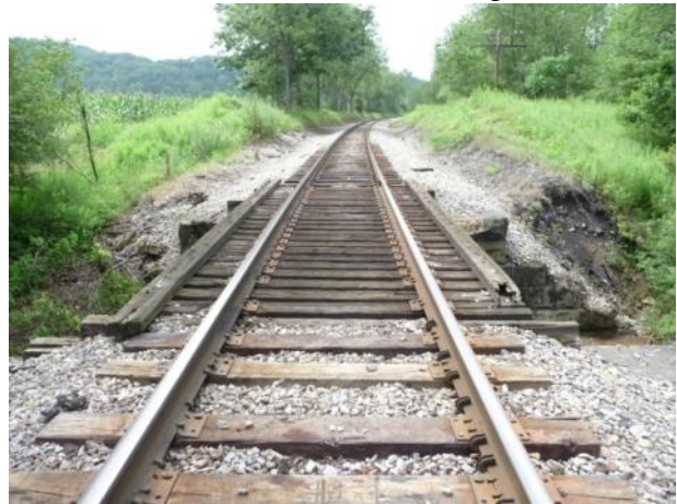
d) Bridge Deck (MP ahead)
