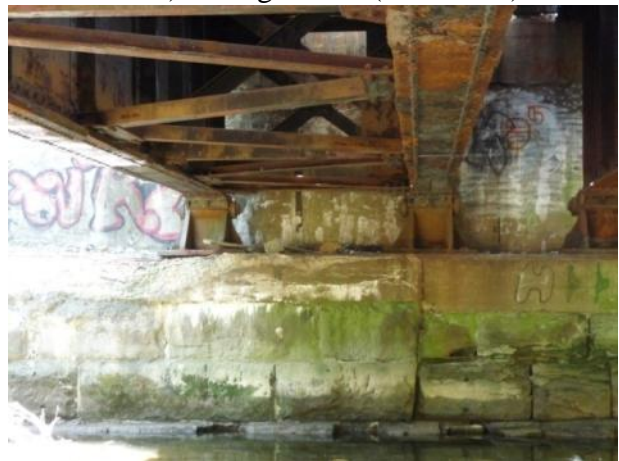
d) Abutment / Bearings (typical)
