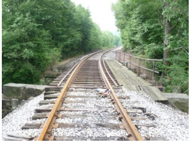
b) Bridge Deck (MP ahead)
