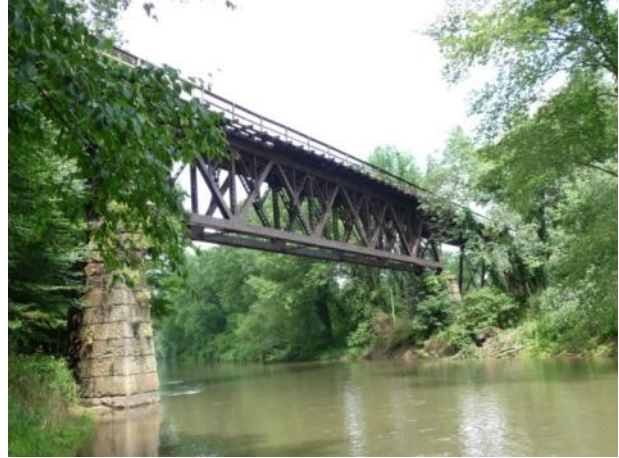
b) View from upstream (right side)
