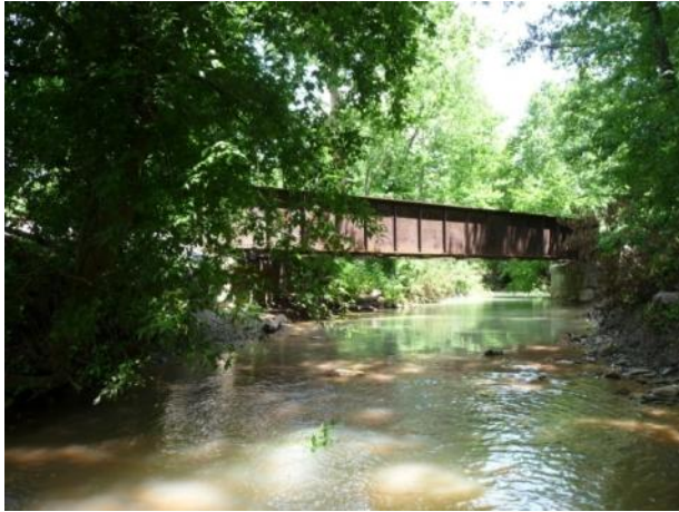
a) View from downstream (right side)
