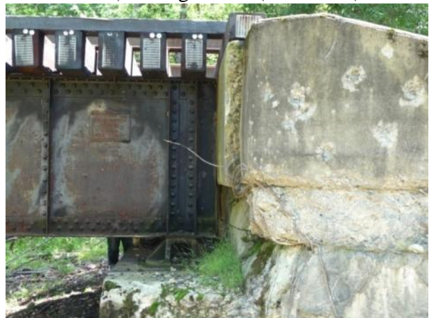
d) Far Abutment / Backwall
