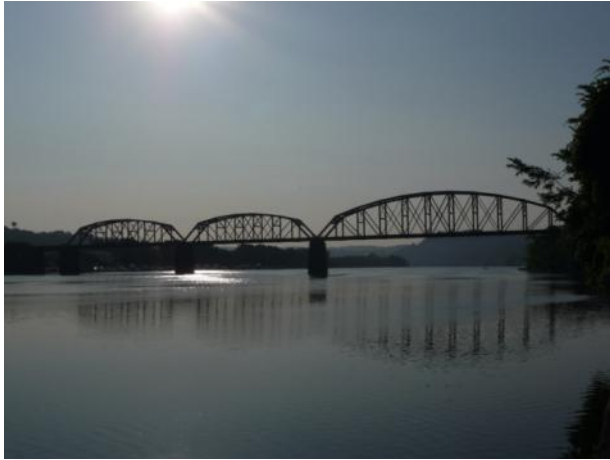
a) View from downstream (left side)
