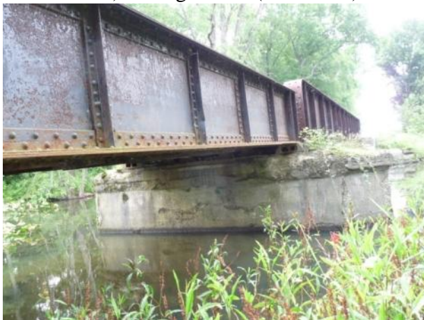
c) Right side (Span 1)
