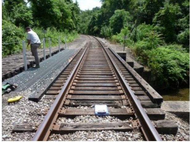
b) Bridge Deck (MP ahead)
