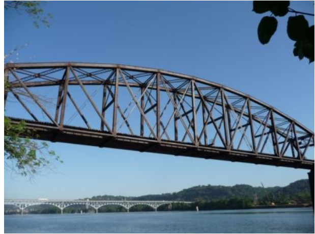
b) View from upstream (right side)
