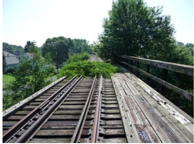
b) Bridge Deck (MP ahead)
