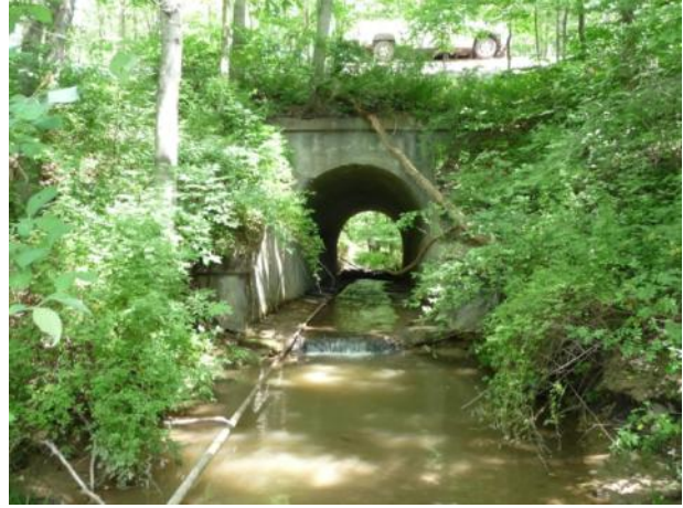
b) View from downstream (right side)
