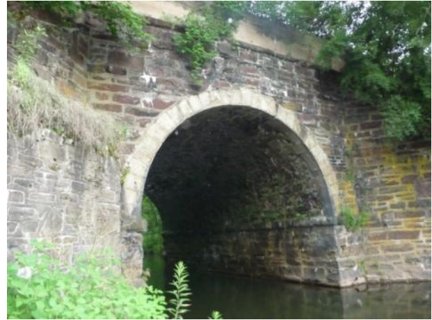
b) View from upstream (right side)
