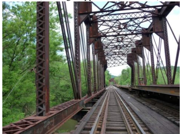
d) Bridge Deck
