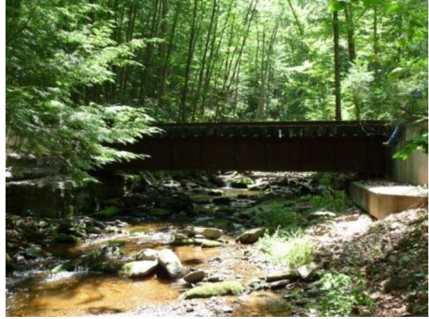
b) View from downstream (right side)
