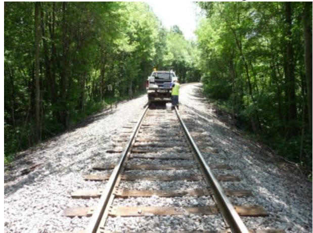
d) Track over (MP ahead)
