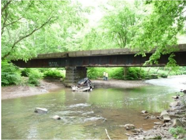
a) View from downstream (left side)
