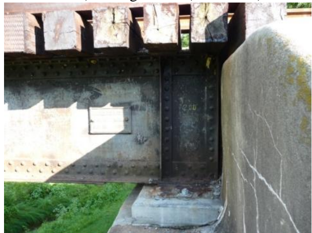
d) Plate Girder / Bridge Seat
