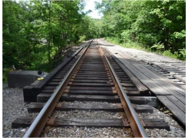
b) Bridge Deck (MP back)
