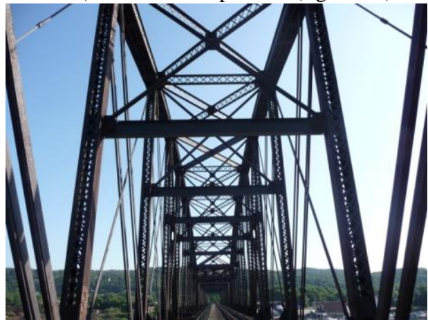
d) Through Truss
