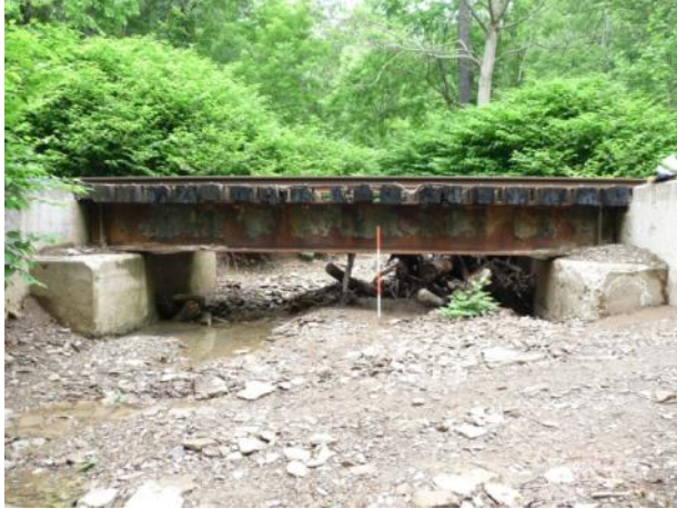
a) View from downstream (right side)
