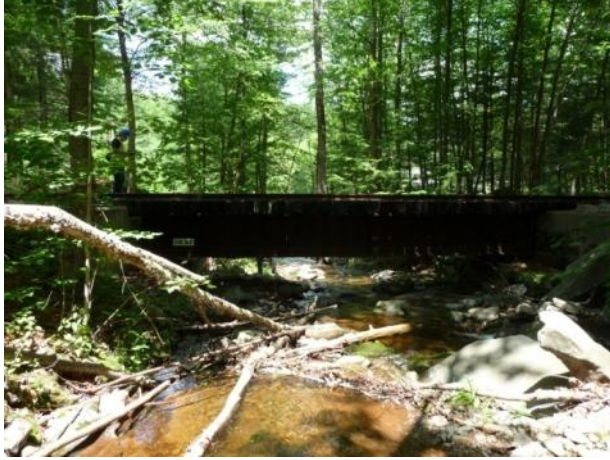
a) View from upstream (left side)
