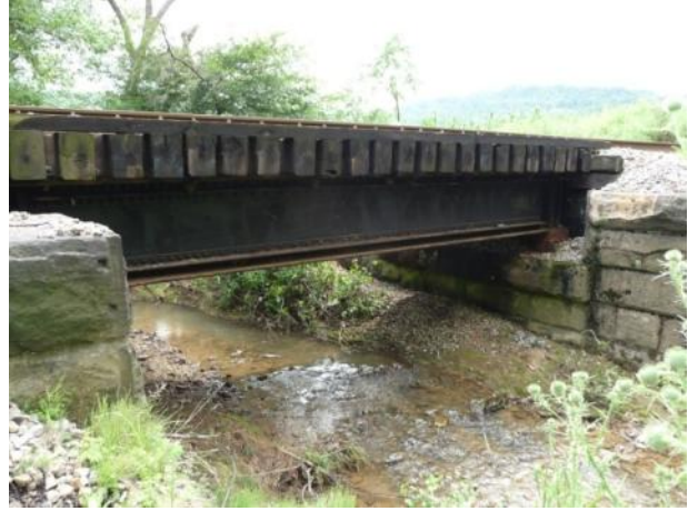
b) View from downstream (right side)
