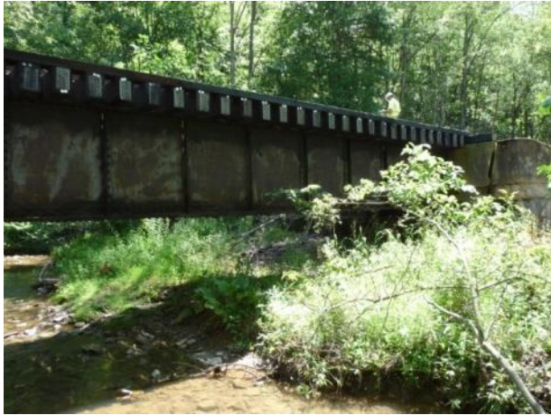
a) View from downstream (right side)
