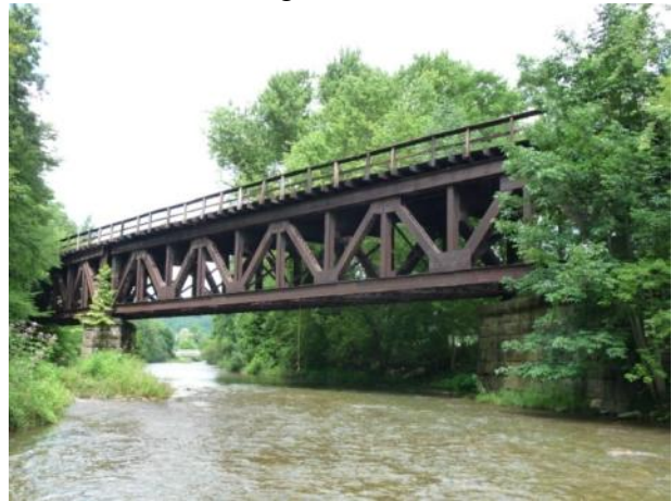
d) View from downstream (span 2)
