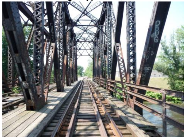
d) Through Truss
