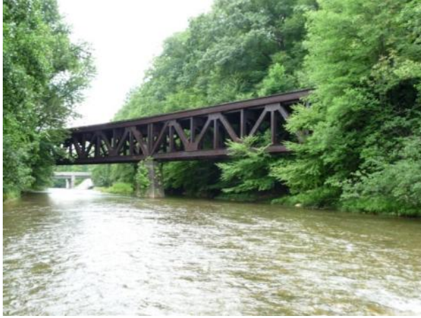
a) View from upstream (left side)
