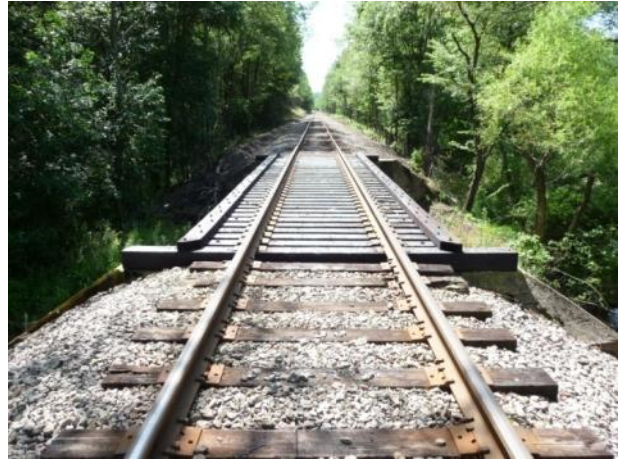
b) Bridge Deck (MP ahead)
