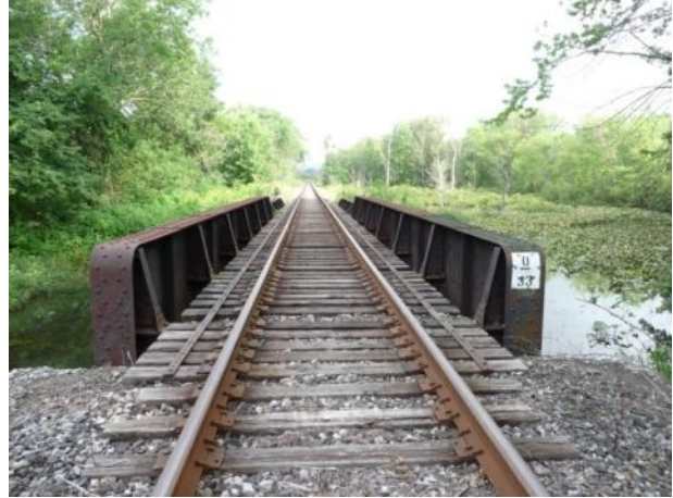
b) Bridge Deck (MP back)
