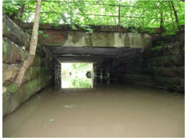
b) View from downstream (right side)
