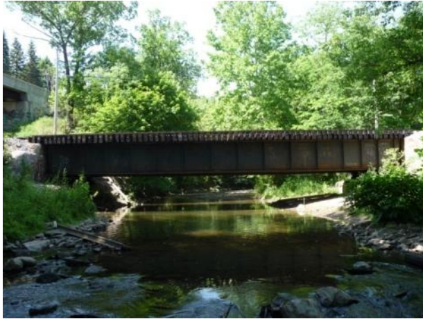
a) View from downstream (right side)
