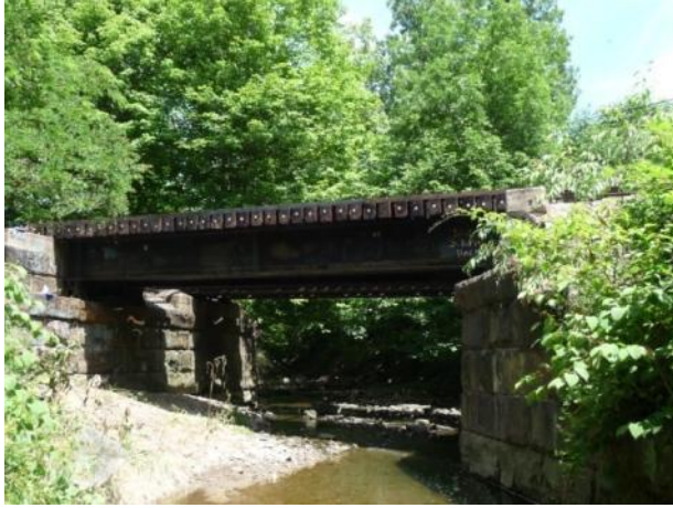
a) View from downstream (right side)
