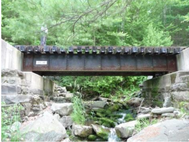
a) View from downstream (right side)
