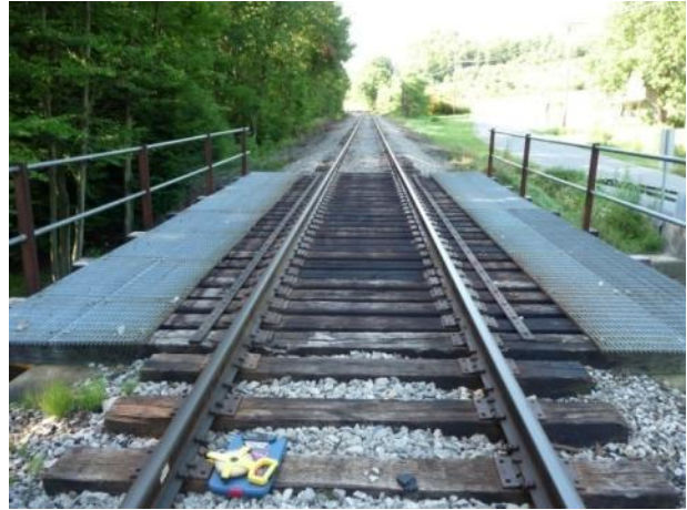
b) Bridge Deck (MP ahead)
