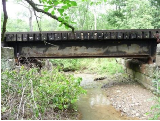
a) View from upstream (left side)
