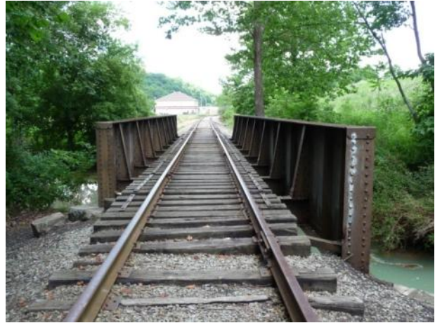
b) Bridge Deck (MP back)
