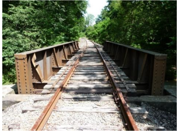
b) Bridge Deck (MP ahead)
