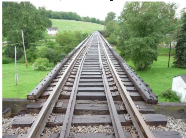
d) Bridge Deck (MP back)
