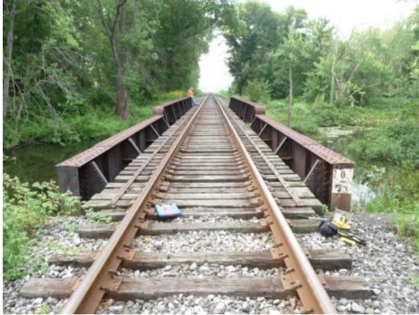
a) Bridge Deck (MP ahead)
