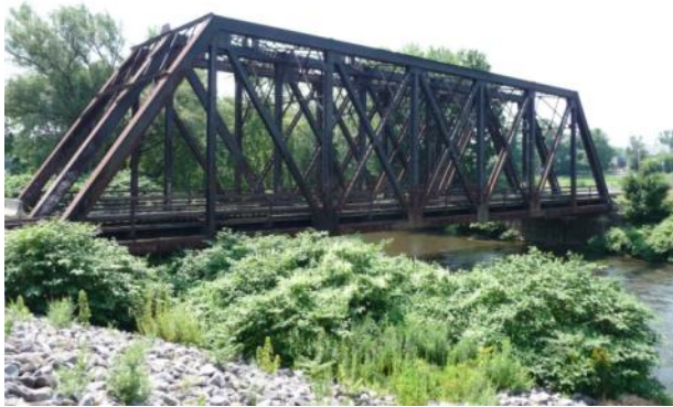
a) View from downstream (left side)
