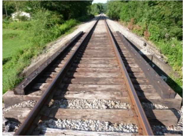
b) Bridge Deck (MP ahead)
