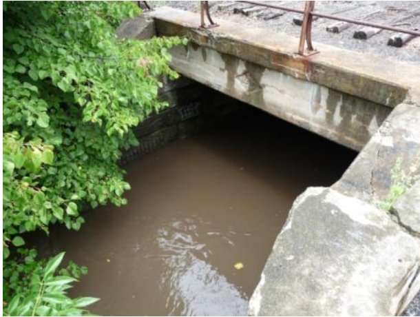
a) View from upstream (left side)
