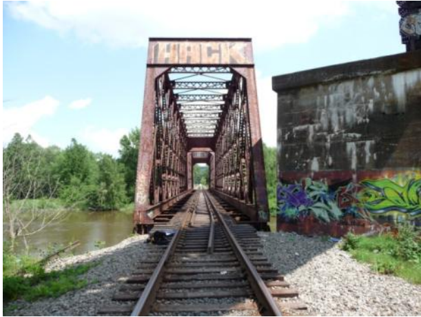
a) Bridge Approach (MP ahead)
