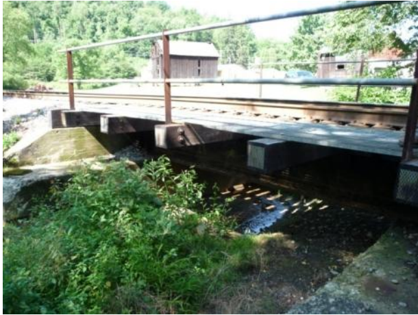
a) View from downstream (left side)
