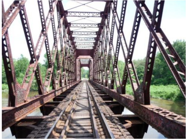
b) Bridge Deck
