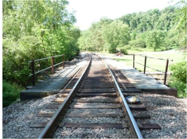
b) Bridge Deck (MP ahead)
