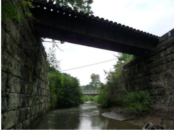
a) View from downstream (left side)
