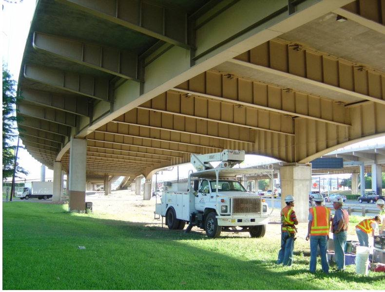
Figure 5.3: Ongoing inspection and maintenance of the structure
