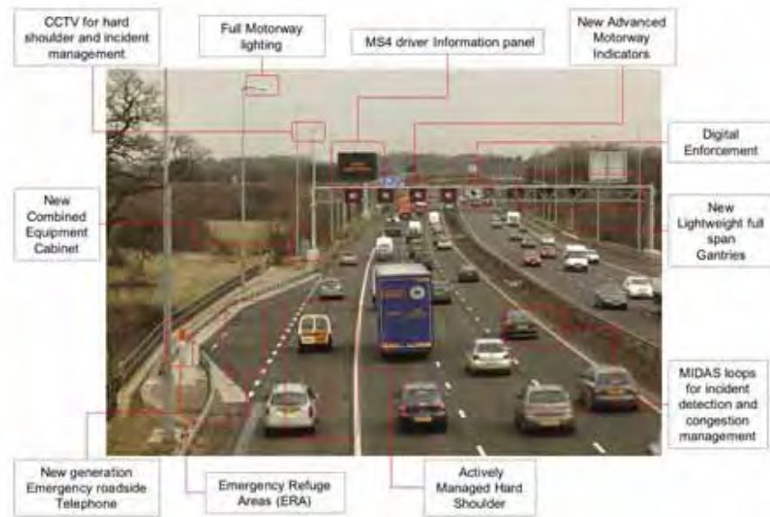
Figure 2.3: Active traffic management on M42
