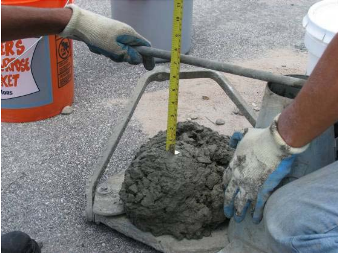
Figure 2.2.12 – Typical Slump Test
