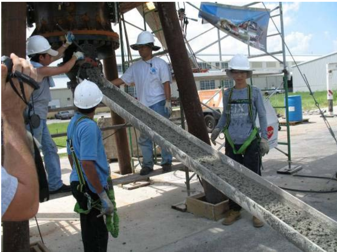
Figure 2.2.14 – Evacuation of concrete from the rocket
