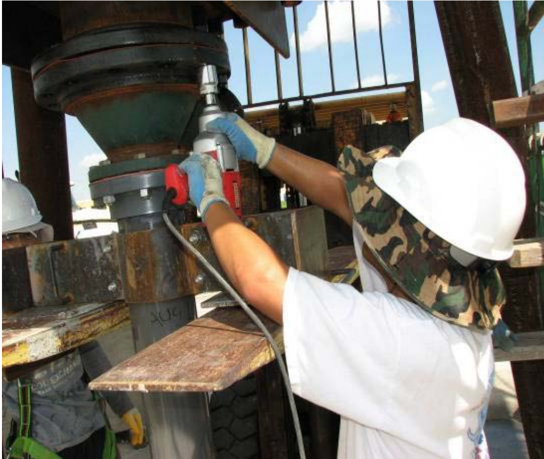
Figure 2.2.20 - Removing the concrete filled clear PVC pipe with an impact wrench
