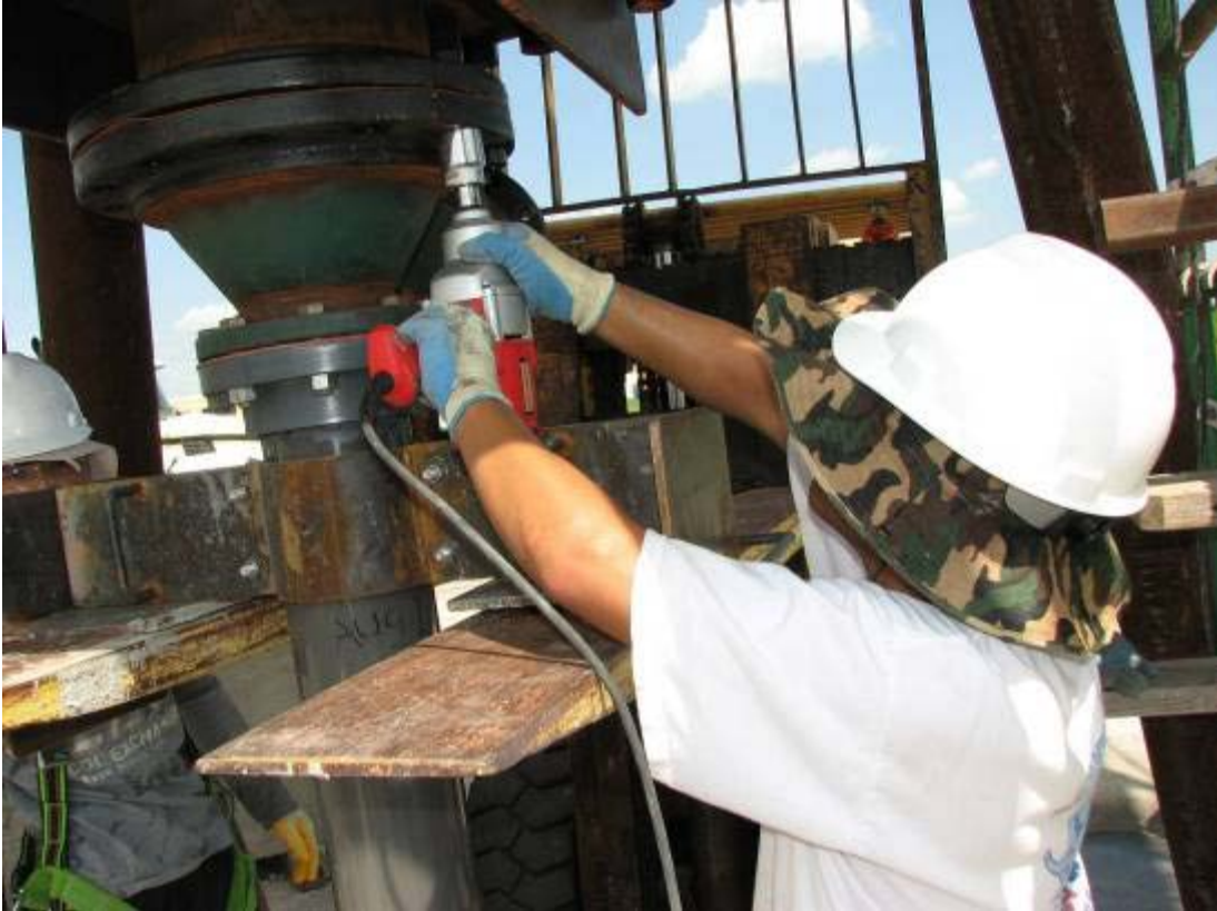
Figure 2.2.10– 6” Clear PVC pipe attached through a reducer
