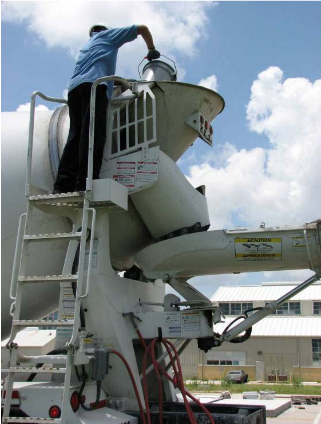
Figure 2.2.11 – Addition of retardant in the concrete truck
