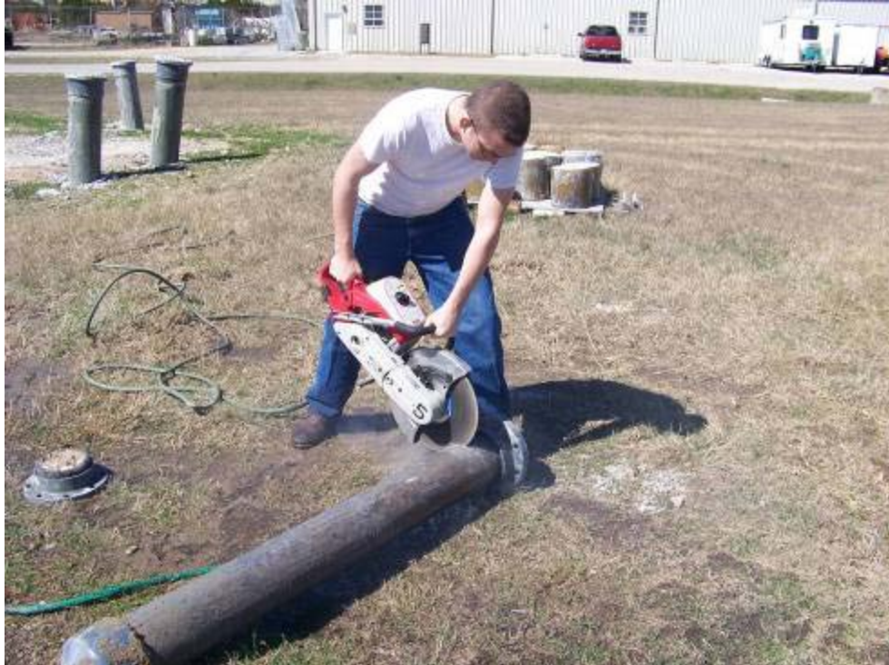
Figure 2.4.1 – Cutting the PVC pipe
