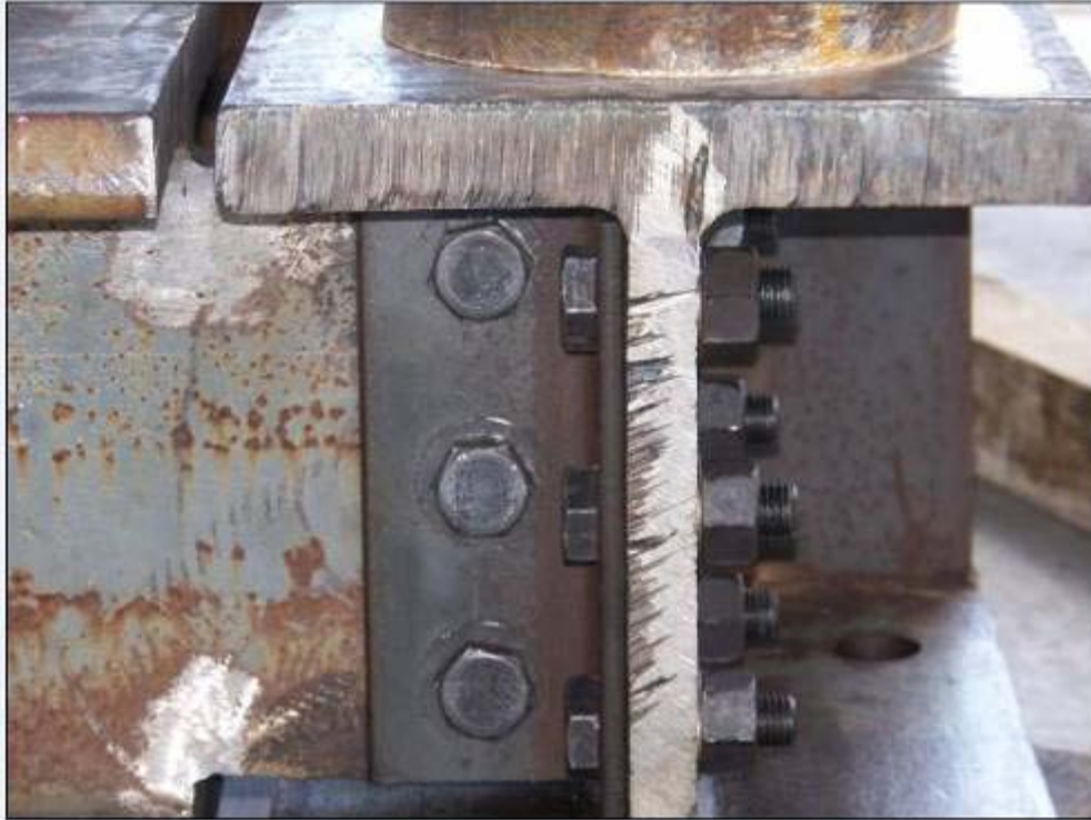
Figure 2.3.17 – Double angle shear connection between beams
