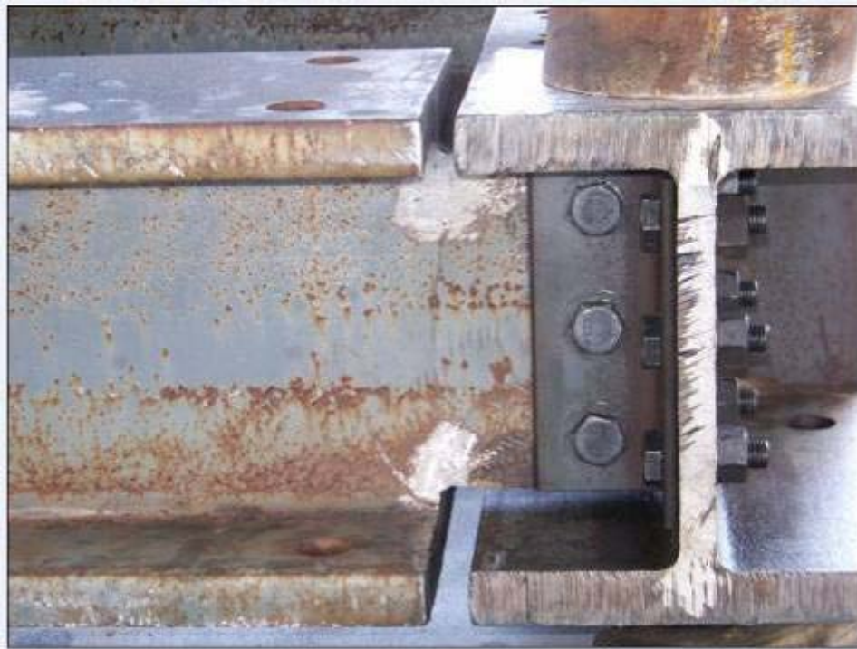
Figure 2.3.18 - Double angle shear connection between beams
