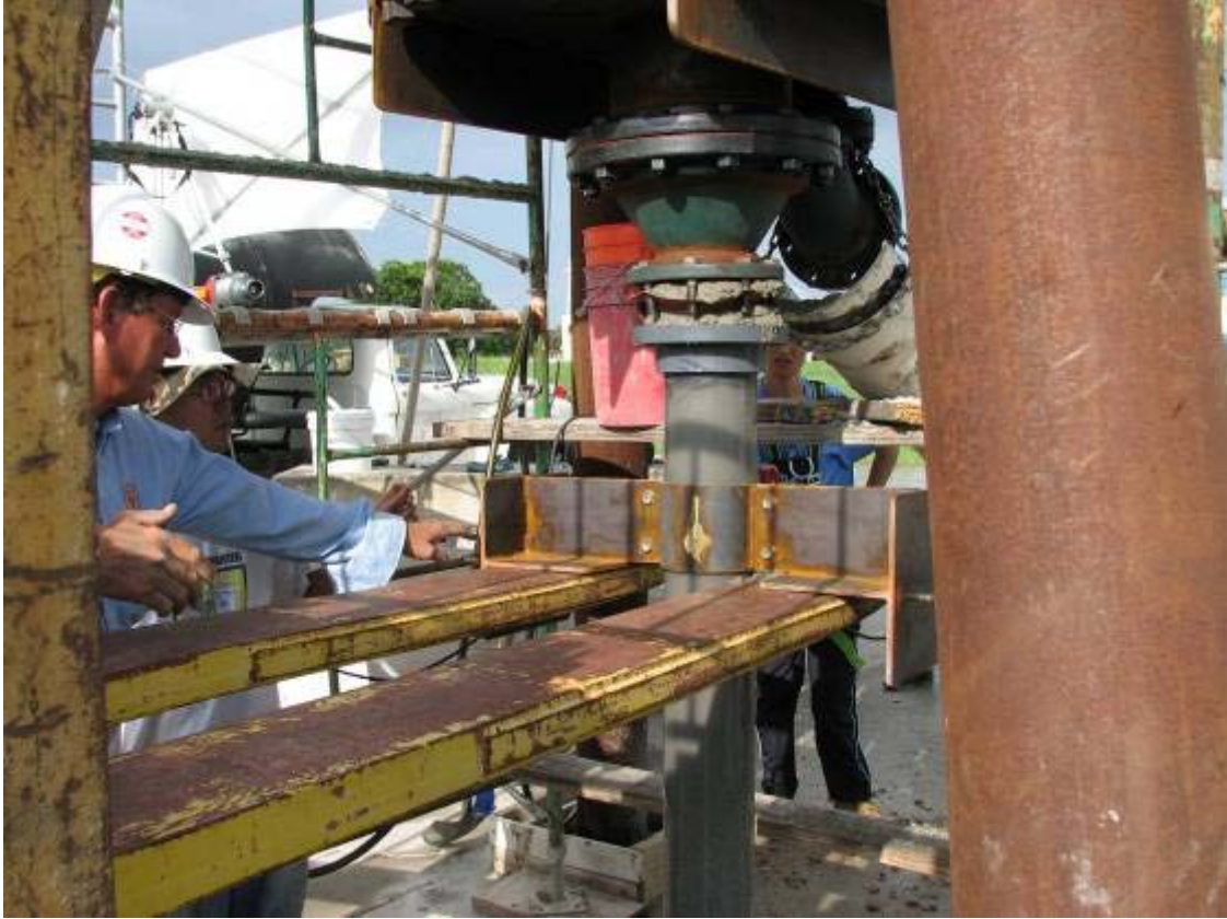
Figure 2.2.21 – Clamps holding PVC pipes to enable their movement with forklift
