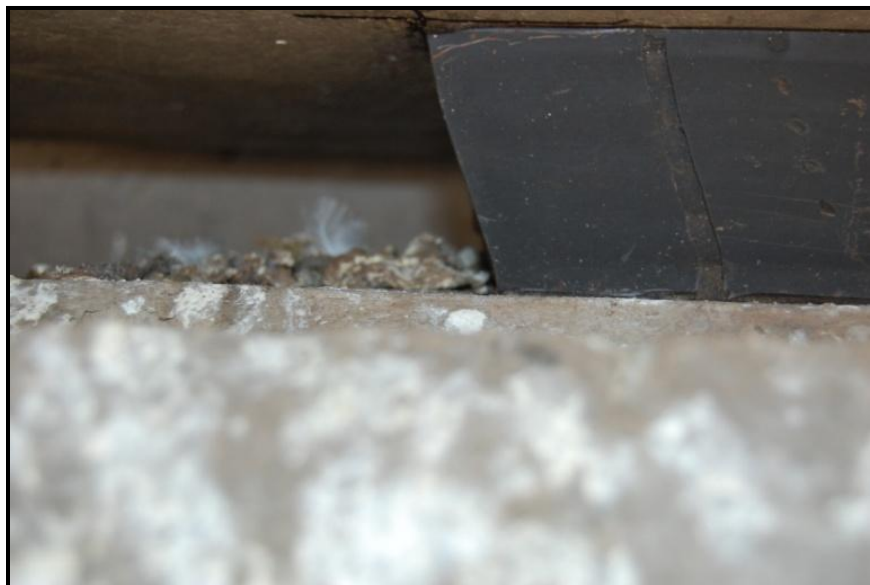
Figure 4.3 – Close-up of Bearing C
