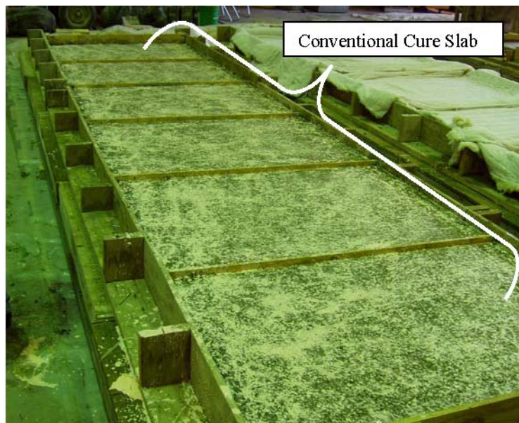
Figure 4.7 Conventional Slab with Curing Compound Prior to Wet Mat Placement
