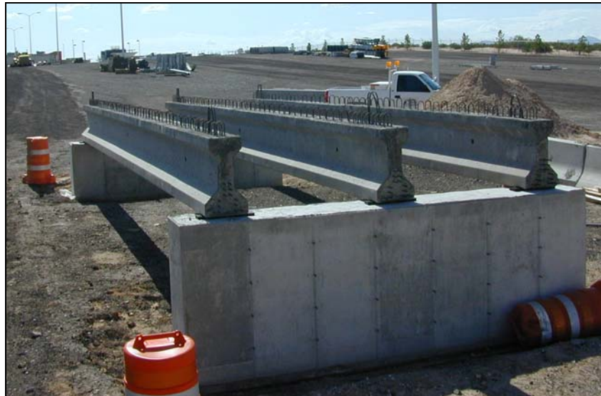
Figure 2.3 Placed Concrete Beams on Abutment Walls
