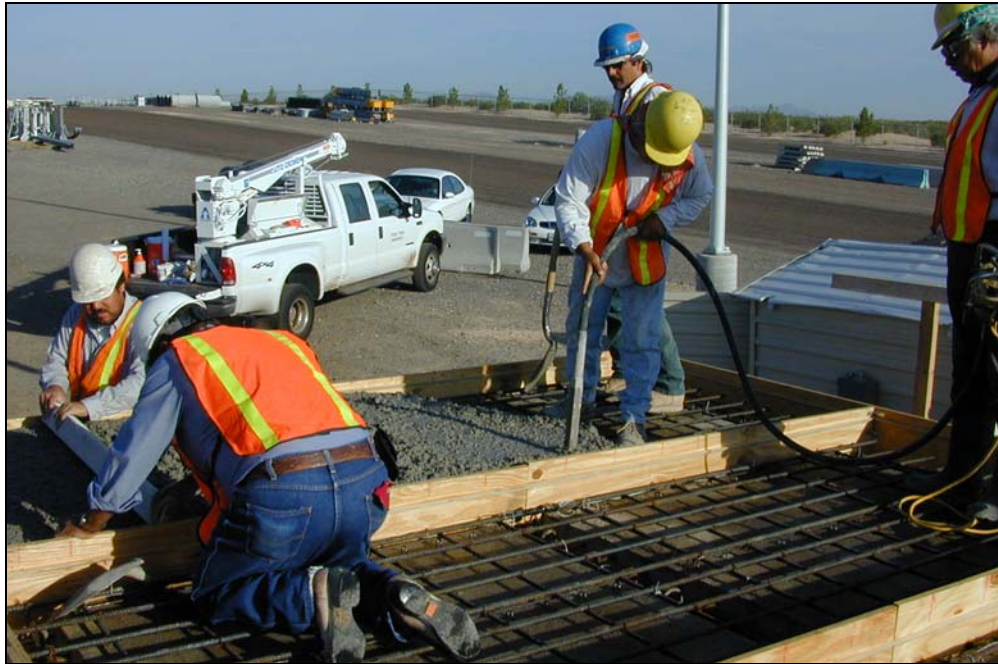
Figure 2.9 Placement of Concrete
