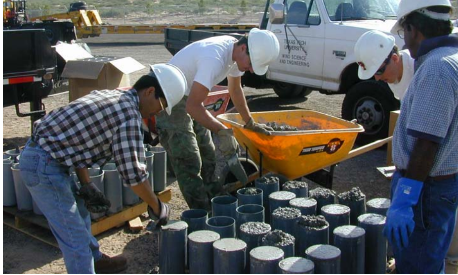
Figure 2.12 Preparing Field Cast Cylinders
