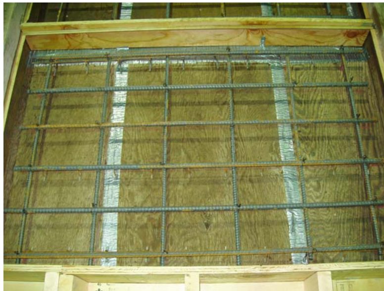
Figure 4.2 Rebar Layout of Slab Arrangement in Structures Laboratory
