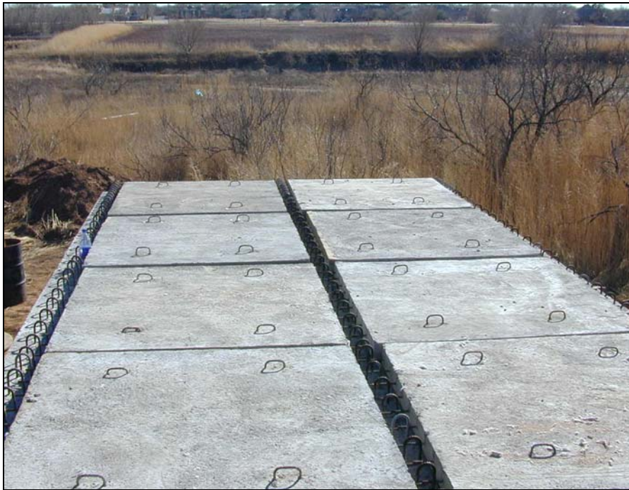
Figure 2.5 Placed Pre-cast Panels on Bridge Deck (Double Bay)
