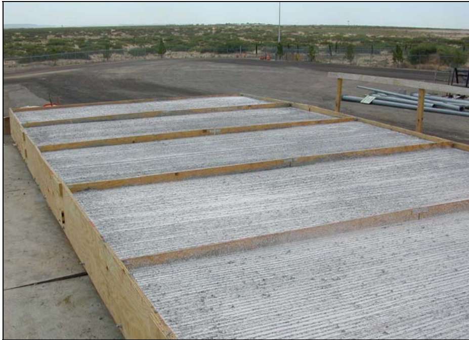
Figure 2.10 Freshly Poured Deck with Finish and Curing Compound
