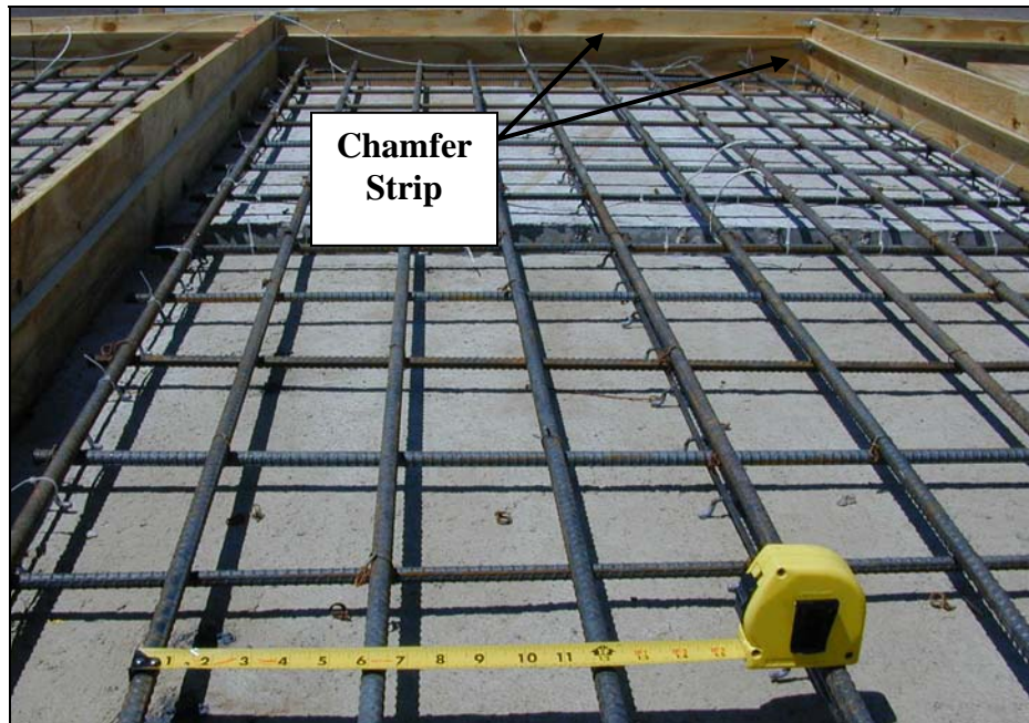
Figure 2.6 Rebar Mat in One Section of the Bridge Deck (Double Bay)
