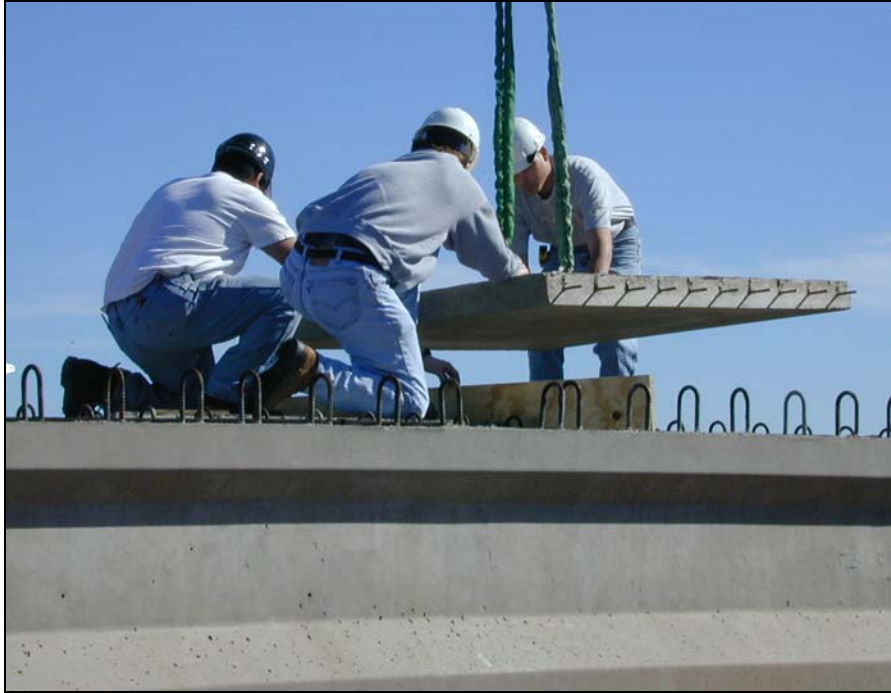
Figure 2.4 Placing Pre-cast Panels on Beams
