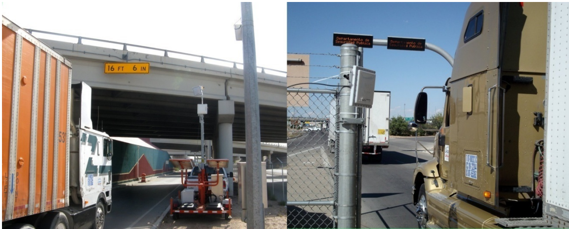
Figure 51. Set up of RFID Stations on Day 2 at Entrance and Exit of the DPS Facility.
