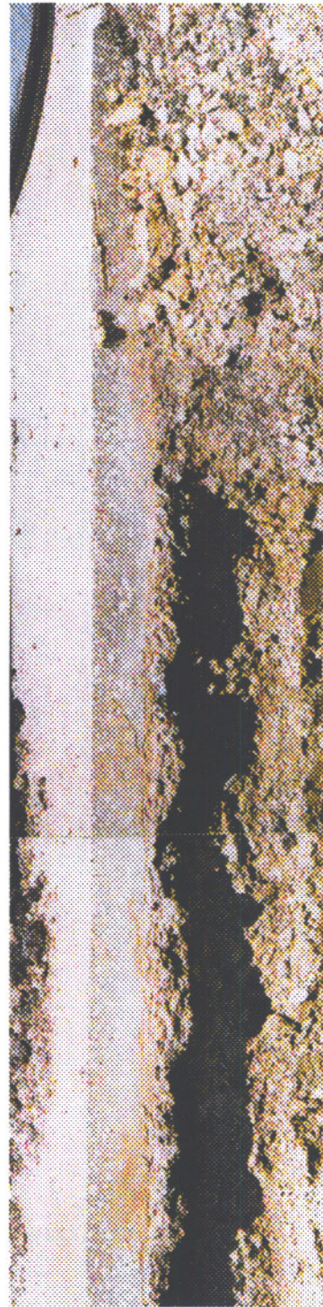
Figure 49 Trench at Station 1+50 Section 390101
