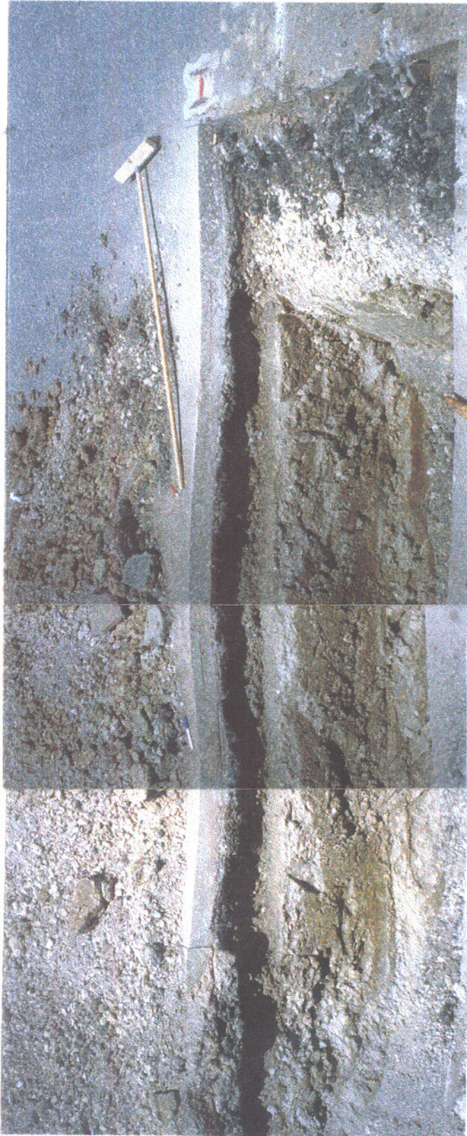
Figure 51 Trench at Station 2+65 Section 390101
