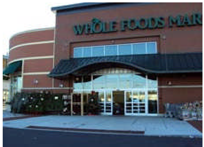
The Whole Foods Market in Denham, Massachusetts uses a 400 kW fuel cell power system from UTC Power to provide 90% of the stores electrical needs, and virtually all its hot water.
