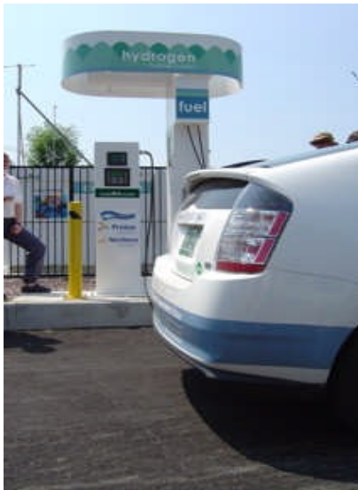
The EVERmont Hydrogen Filling Station opened in Burlington, Vermont in 2006. Hydrogen is produced from wind-powered electrolysis with a Proton Energy Systems electrolyzer.
