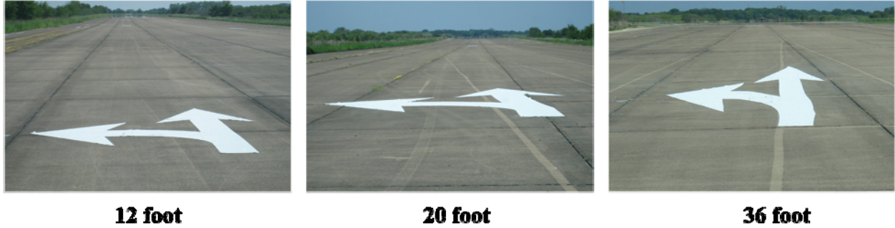
Figure 28. “Left and Through” Pavement Marking Symbols.
