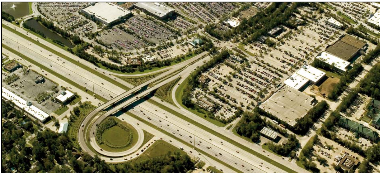
Figure 3. Interchange Added to I-45 Using Multi-Partner Funding.
