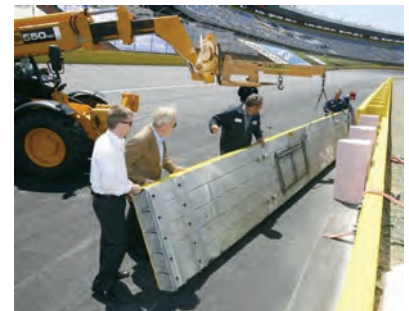
The MwRSF's SAFER barrier uses foam cushioning to make racetrack guardrail impacts safer. Indy Racing League Senior Technical Director Phil Casey has called it "the greatest achievement for safety in automobile racing that's been made."
