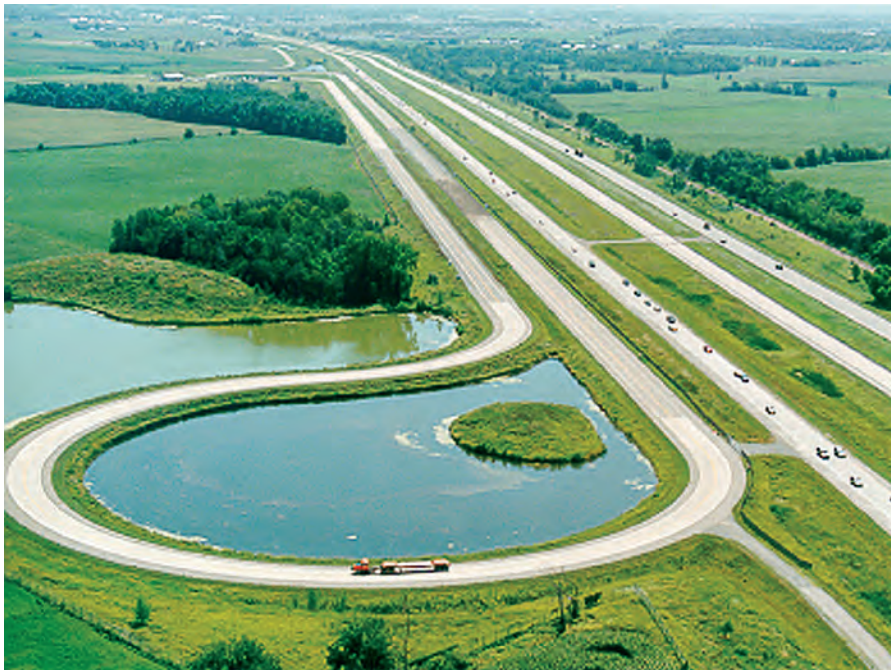
SP&R funding provides increased opportunities to use the MnROAD cold-region testing laboratory, a unique platform for testing road-building materials and designs. MnROAD features two road segments—3.5 miles of mainline highway and 2.5 miles of low-volume roadway—divided into 52 test cells.
