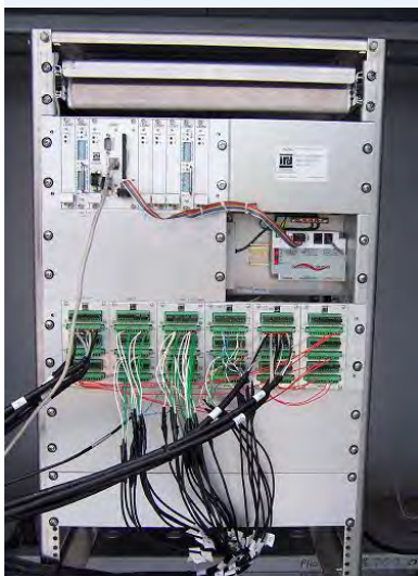
This controller is an example of those used at Mn/DOT's WIM sites.
