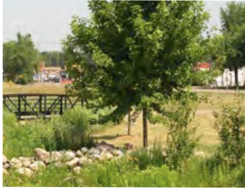
Bioretention facilities use natural processes to control stormwater overflow and filter pollutants.
