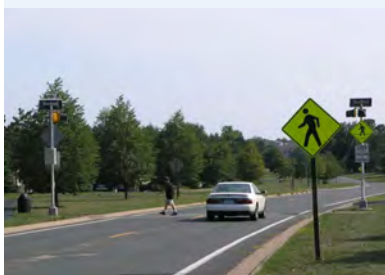
Researchers studied user-activated warning crosswalks such as this one in Woodbury, Minnesota.
