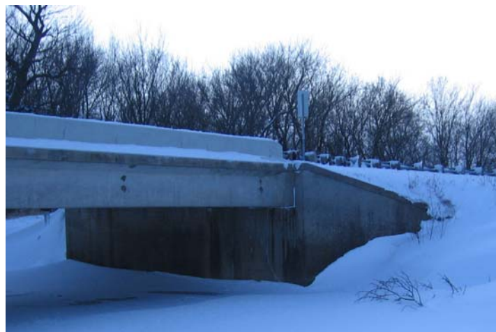
Figure 7.2: Bridge 6468 - upstream left abutment
