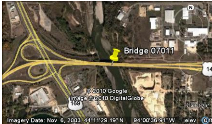
Figure 7.10: Bridge 07011 - aerial view from Google Earth
