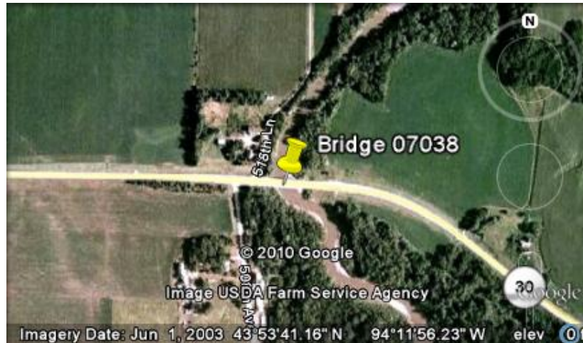
Figure 7.14: Bridge 07038 - aerial view from Google Earth
