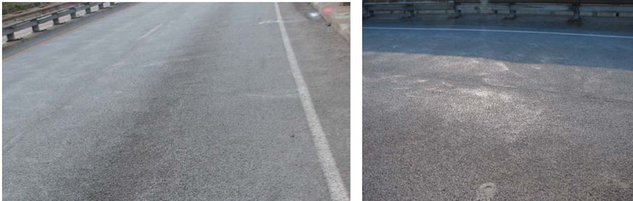
Figure 4.4. Photographs showing general overall integrity of the Hibbing SafeLane™ installation after two years (left: September, 2008) and three years (right: July, 2009).
