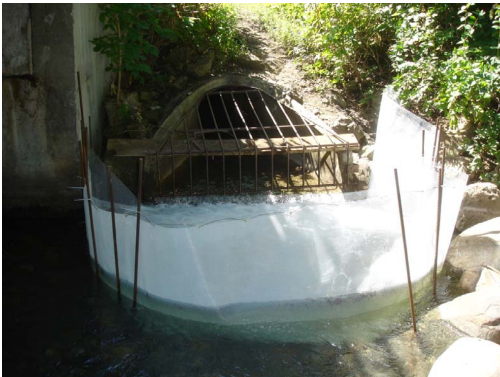
Figure A-5: Sediment capture screen at Rice Creek
