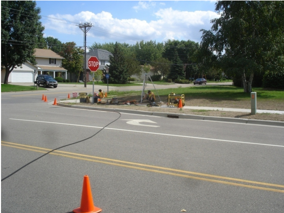
Figure A-6: Field site with confined space entry tripod
