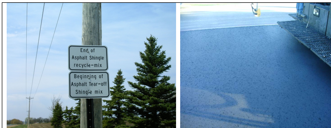
Figure 5.7. Hennepin County Rd. 10 RAS Construction
