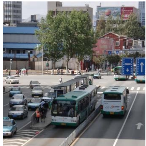
Kunming Busway, Station, and Typical Vehicles
