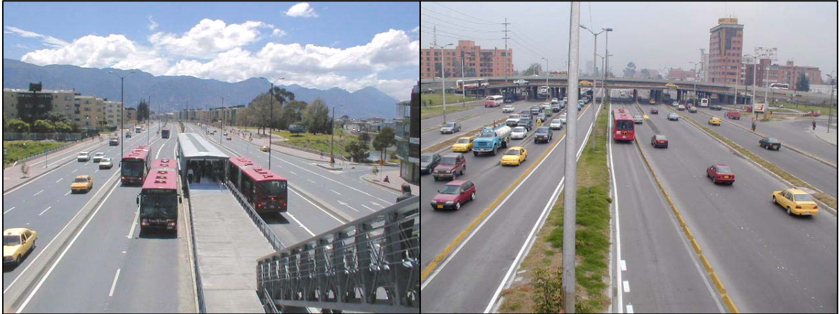
FIGURE 2.7 – Dual and Single Carriageways
